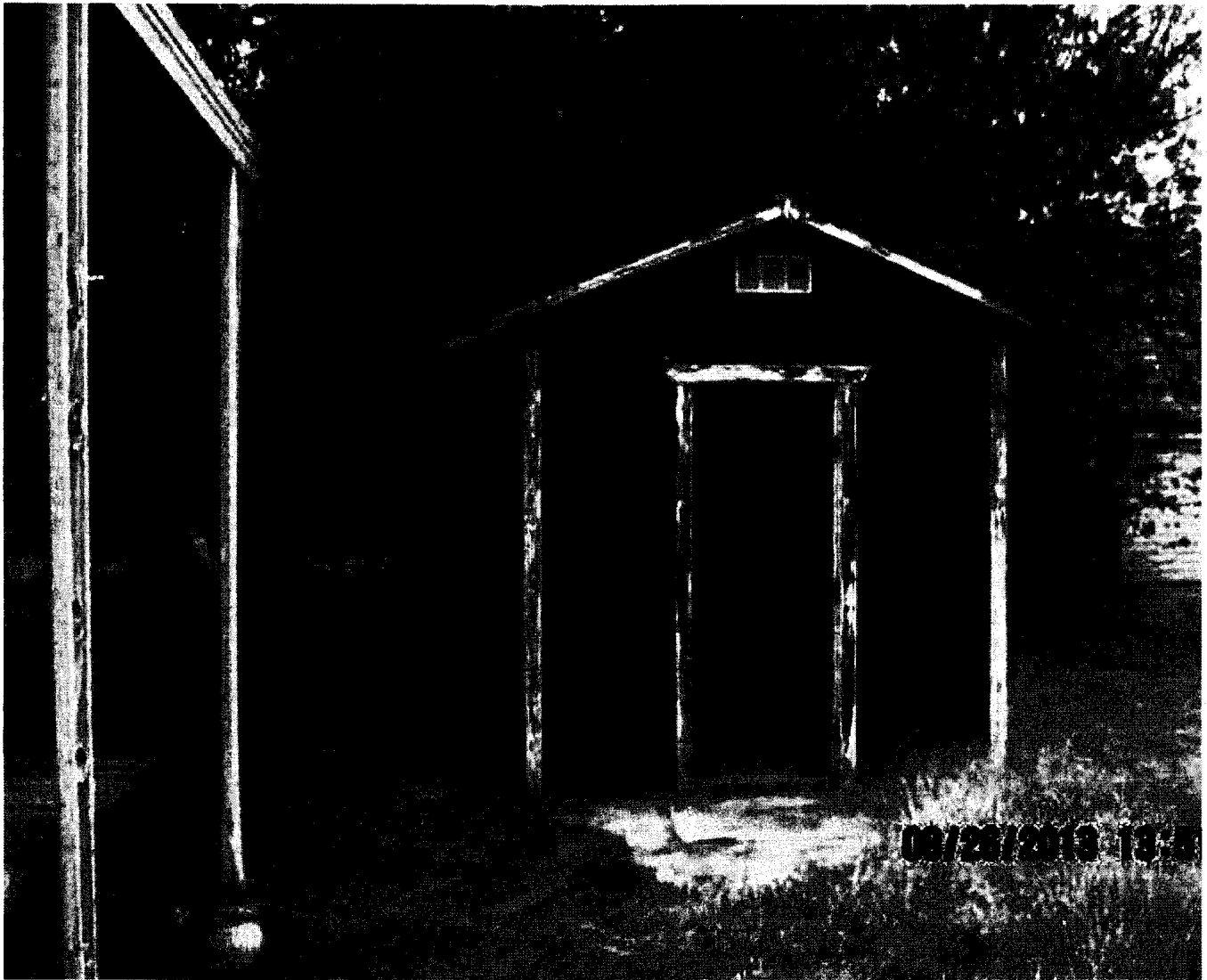
E. Torres; substandard shed defects- 12, 13, 14, 17 - 08/26/2013
