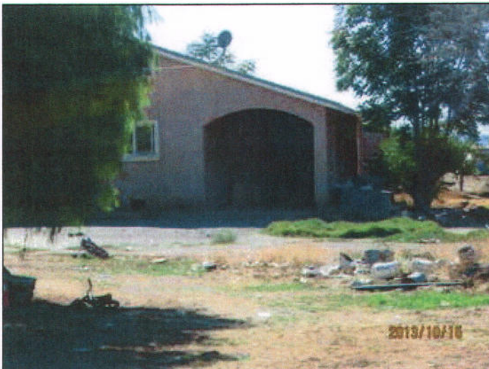
10/15/13 Rubbish and discarded debris remain. L Lyon
