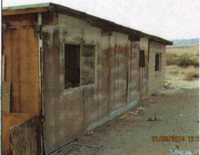
Exterior Wall (North Side) 1/9/14 J. Cole
