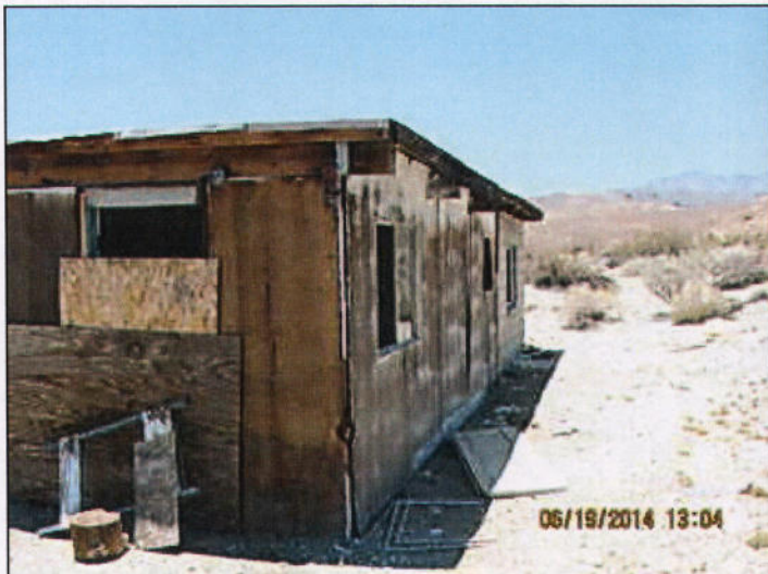
Northeast Corner of the Structure 6/19/14 J. Cole
