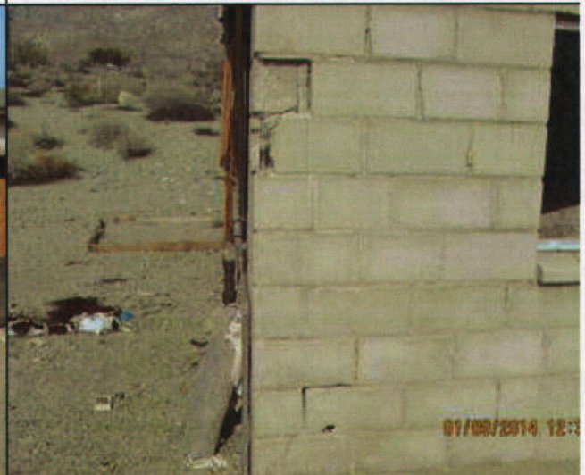
Exterior, Southwest Corner 1/9/14 J. Cole
