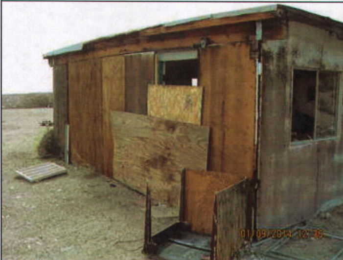
Exterior Wall (East Side) 1/9/14 J. Cole
