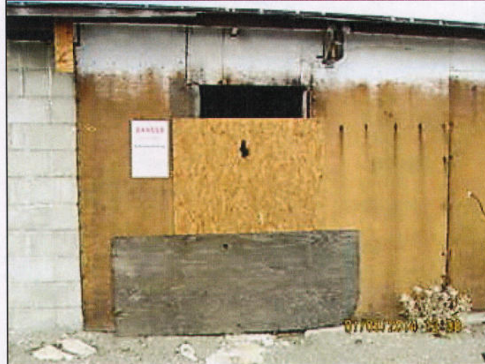
Exterior Wall/Door (North Side) 1/9/14 J. Cole
