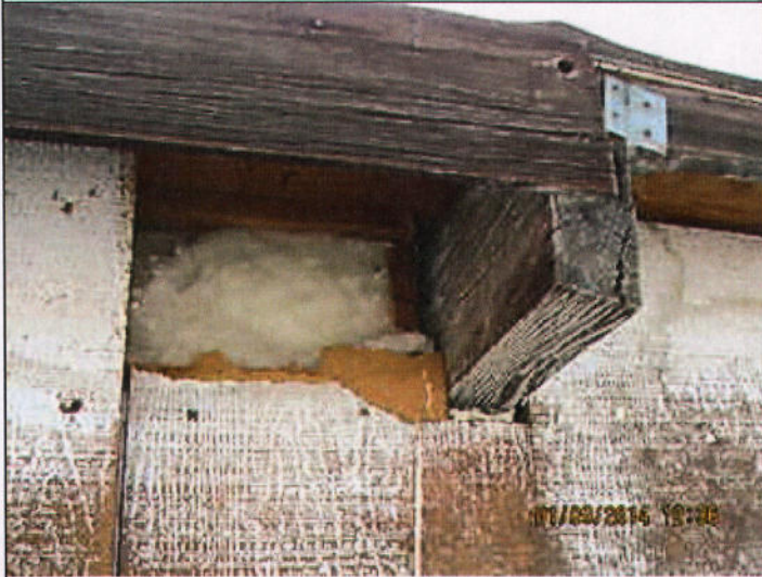
Roof Beam and Exterior Wall 1/9/14 J. Cole
