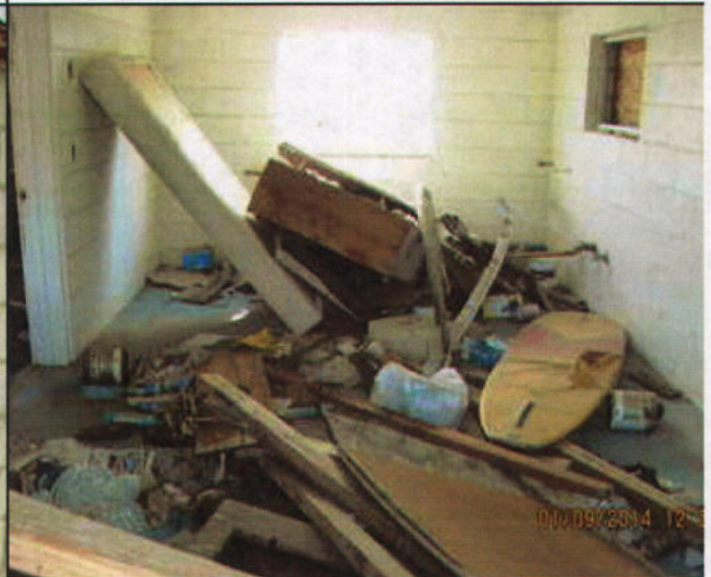
Inside the Structure 1/9/14 J. Cole
