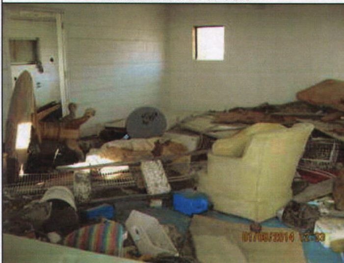
Inside the Structure 1/9/14 J. Cole
