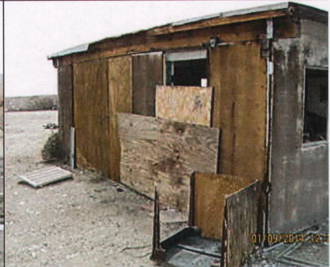
Exterior Wall (East Side) 1/9/14 J. Cole
