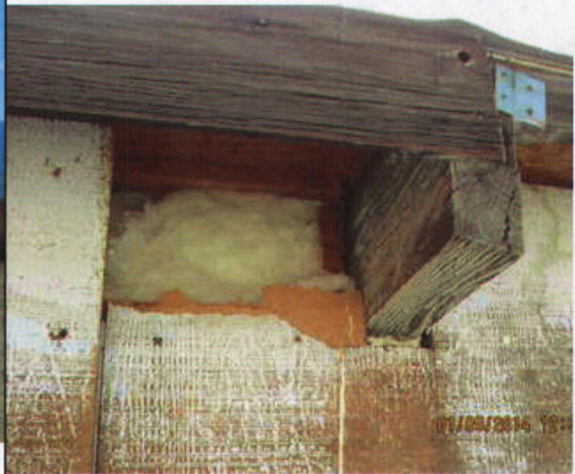
Roof Beam and Exterior Wall 1/9/14 J. Cole
