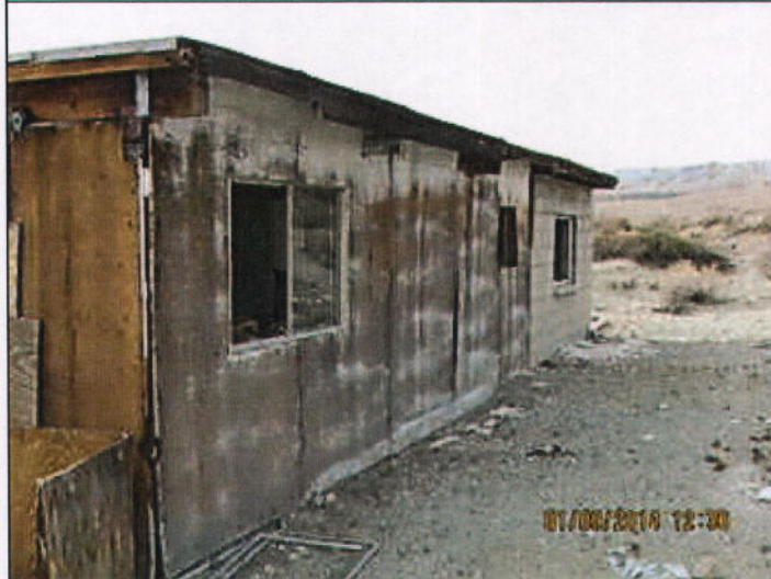
Exterior Wall (North Side) 1/9/14 J. Cole
