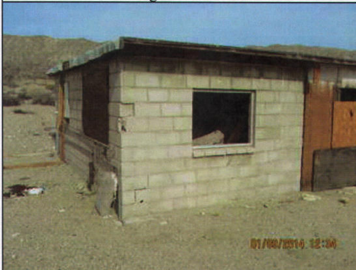
Exterior, Southwest Corner 1/9/14 J. Cole
