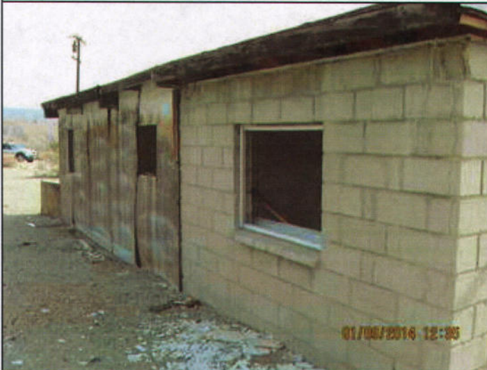
Exterior Wall, North Side 1/9/14 J. Cole
