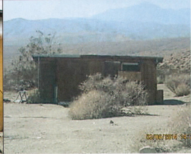
Substandard Structure and Rubbish 3/6/14 J. Co
