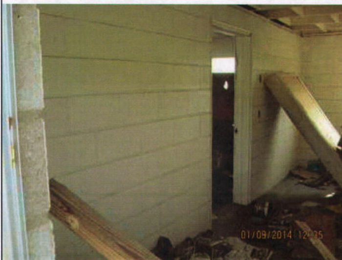
Inside the Structure 1/9/14 J. Cole
