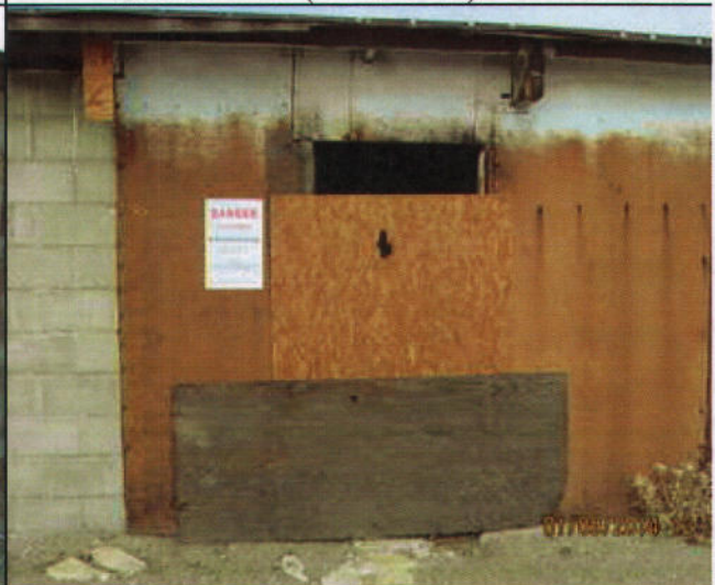
Exterior Wall/Door (North Side) 1/9/14 J. Cole
