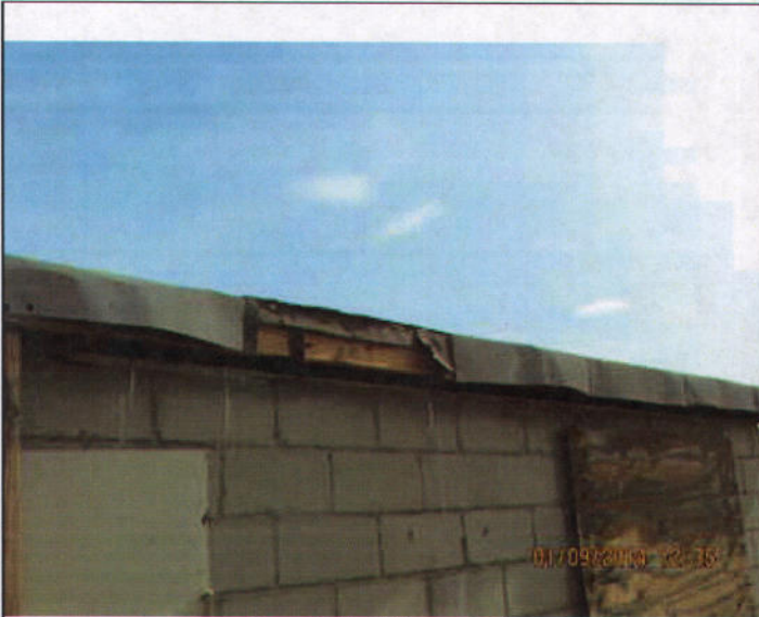
Roof 1/9/14 J. Cole
