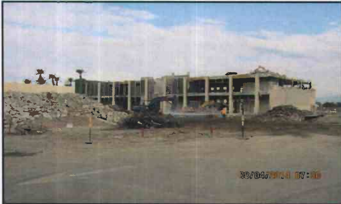
Figure 1. August 04, 2014: Northwest View - CAC Building
