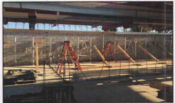
Figure 12. August 29, 2014: Masonry Ramp Wall Bracing with Second Level Deck Scaffolding Beyond
