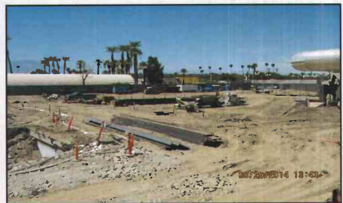
Figure 12. August 29, 2014: Northwest View - Partial Excavation at West Shoring
