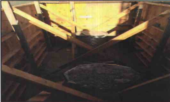
Figure 7. August 26, 2014: Interior of Elevator Foundation Formwork
