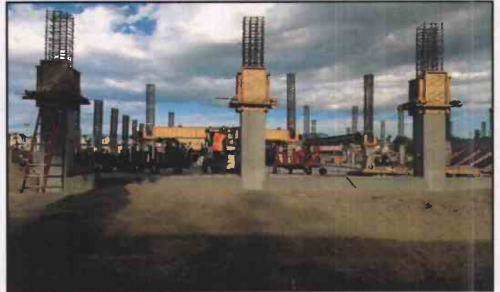
Figure 8. August 26, 2014: Second Level Column Formwork
