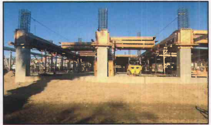
Figure 10. August 29, 2014: Second Level Deck Formwork Placement
