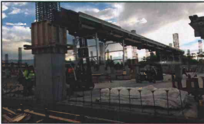
Figure 9. August 26, 2014: Second Level Deck Formwork Scaffolding Placement
