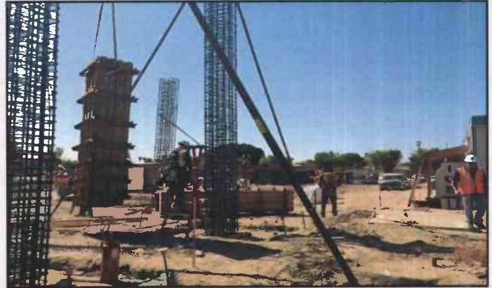
Figure 2. August 14, 2014: Column Form Placement
