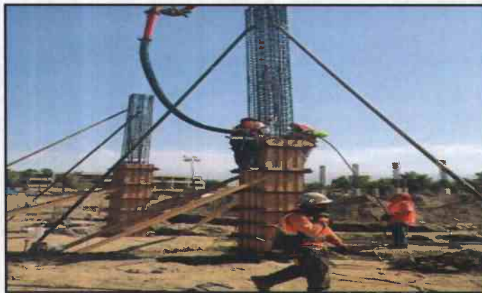
Figure 3. August 12, 2014: Concrete Pour at Columns
