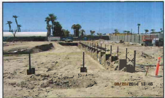
Figure 10. August 29, 2014: West View - North Perimeter Shoring Piles In Place
