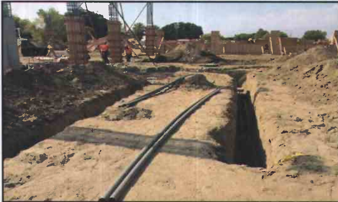
Figure 1. August 12, 2014: IT Data and Telephone Trenches
