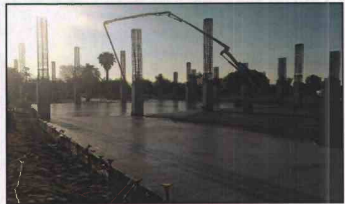
Figure 6. August 22, 2014: Concrete Pour at Slab on Grade
