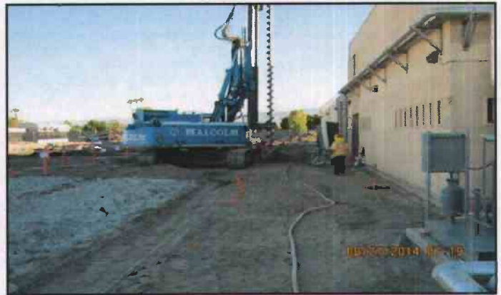
Figure 8. August 27, 2014: Soldier Pile Pre-Drilling for Shoring
