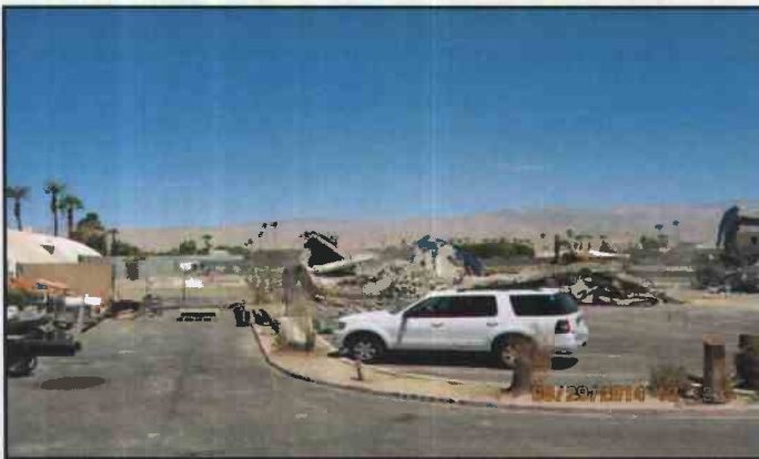
Figure 7. August 29, 2014: North View - CAC Building, Demolished to Grade
