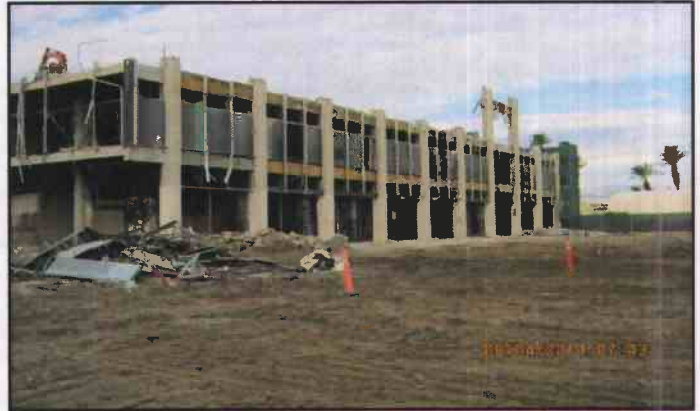
Figure 2. August 04, 2014: Southwest View - CAC Building
