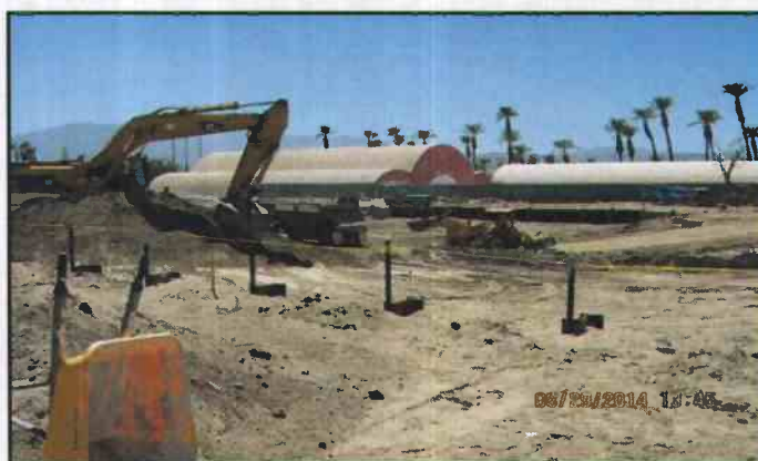
Figure 11. August 29, 2014: Southwest View - East Perimeter Shoring Piles In Place
