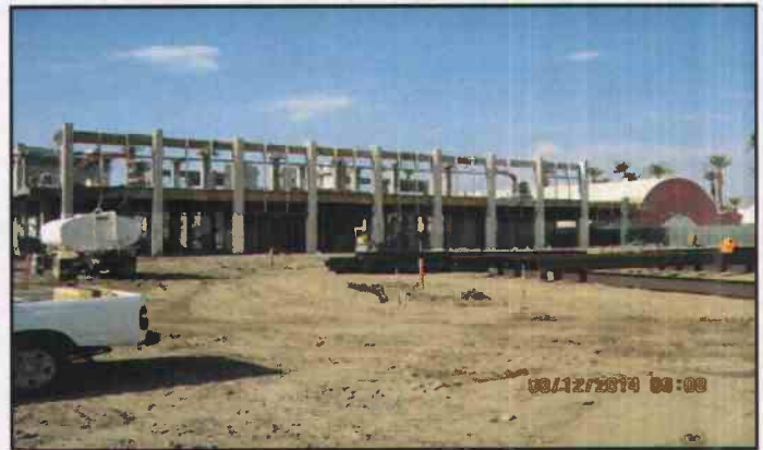
Figure 4. August 12, 2014: South View - CAC Building
