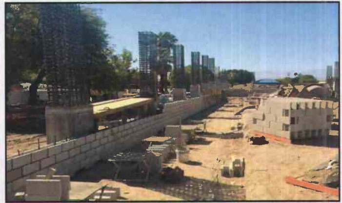
Figure 4. August 14, 2014: Masonry Placement at Driveway/Parking Ramp to Second Level
