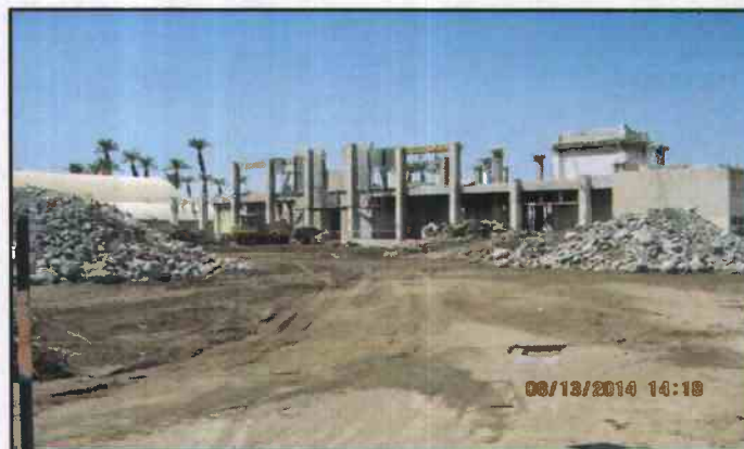
Figure 5. August 13, 2014: Northwest View - CAC Building
