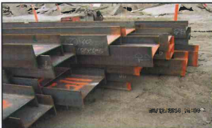
Figure 9. August 12, 2014: Soldier Piles (Wide flange Steel)
