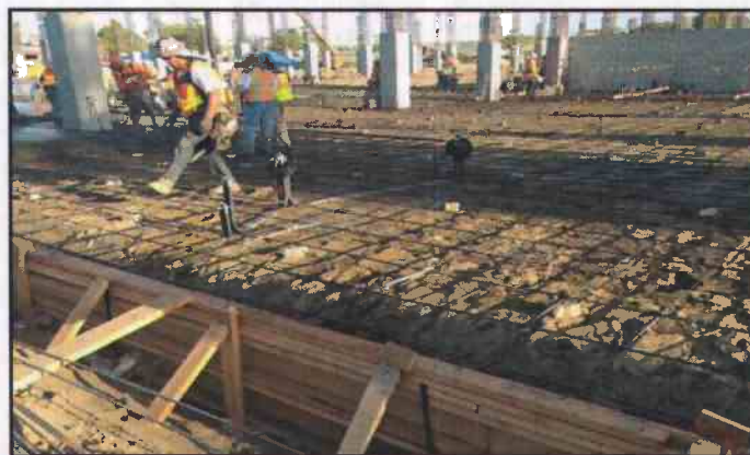
Figure 5. August 22, 2014: Reinforcement Placement at Slab on Grade
