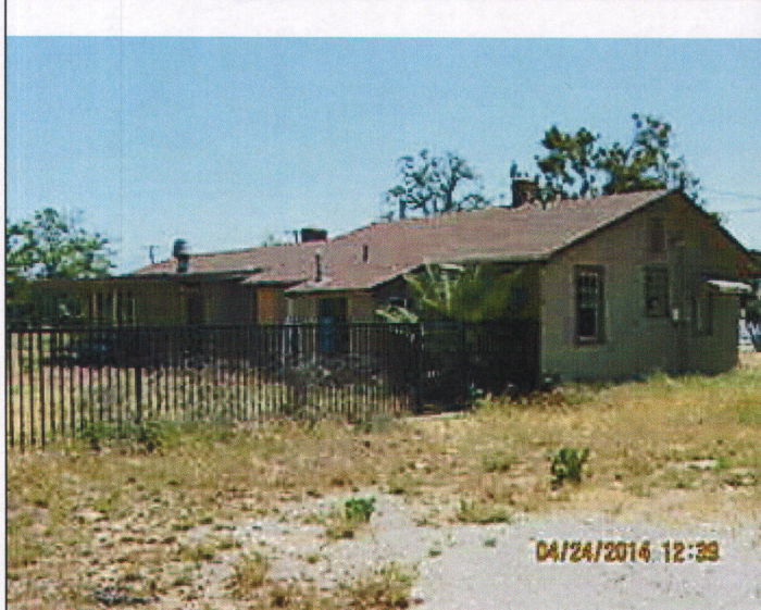
Substandard Structure remains. J. Palmer
