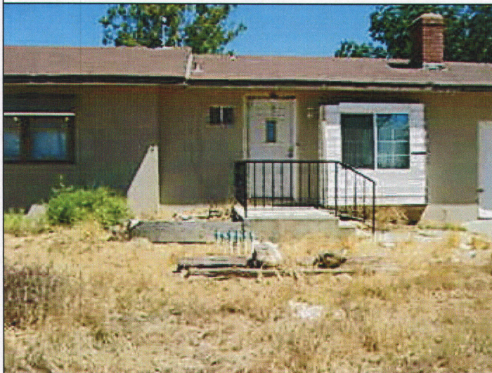
08/09/13 - Substandard Structure NOD# 11,13, 14, 17 - Pike
