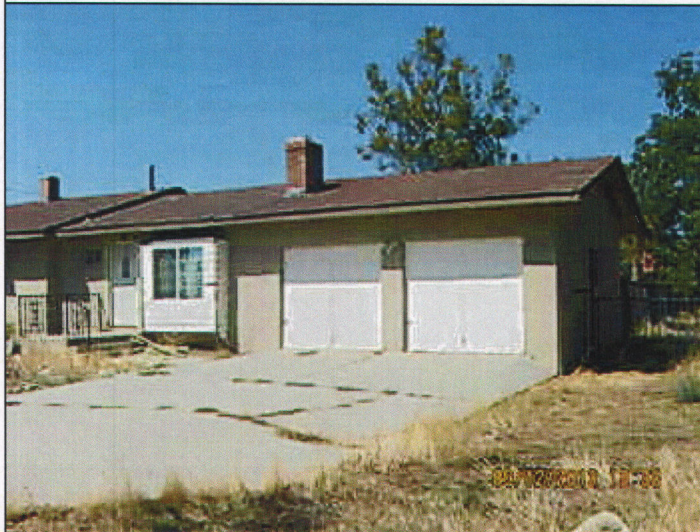
Substandard Structure remains. J. Palmer
