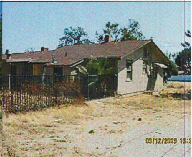
Substandard Structure remains. J. Palmer
