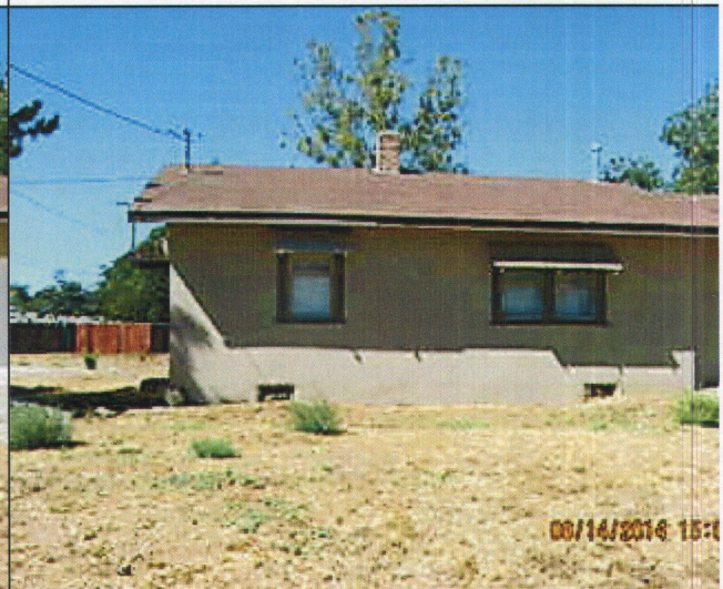
Rubbish removed, Substandard Structure remains. J. Palmer
