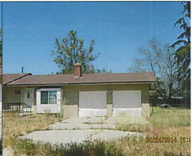
Substandard Structure remains. J. Palmer
