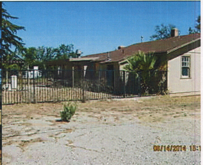
Rubbish removed, Substandard Structure remains. J. Palmer
