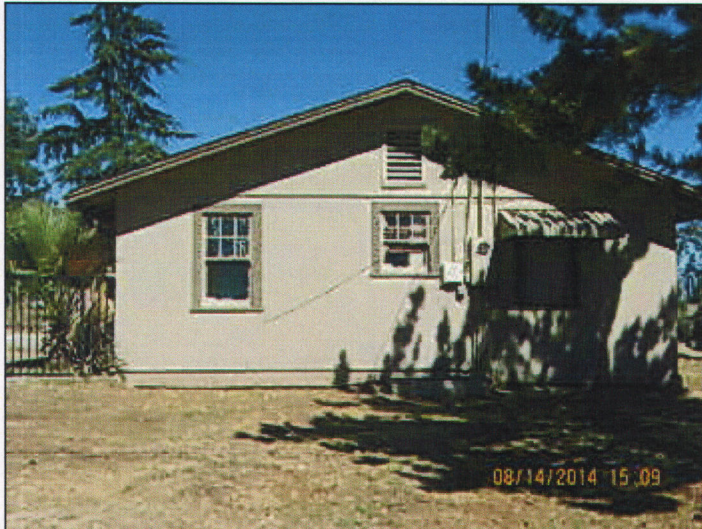
Rubbish removed, Substandard Structure remains. J. Palmer
