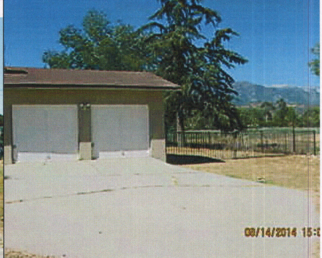
Rubbish removed, Substandard Structure remains. J. Palmer
