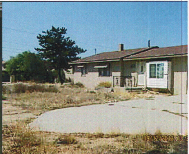
Substandard Structure remains. J. Palmer
