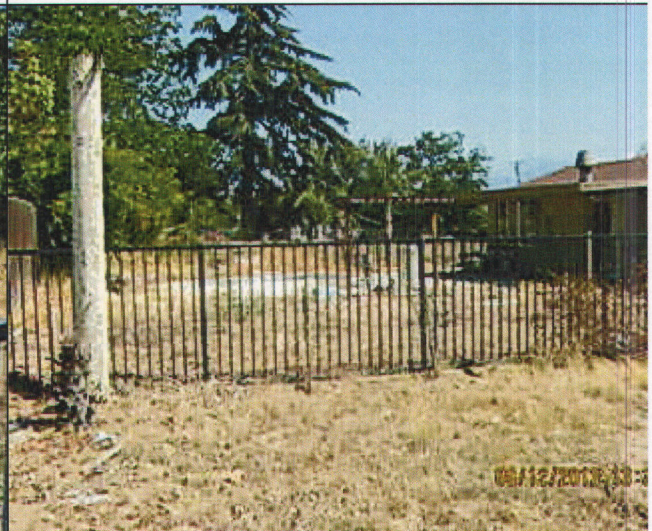
Substandard Structure/Accumulated Rubbish remains. J. Palmer
