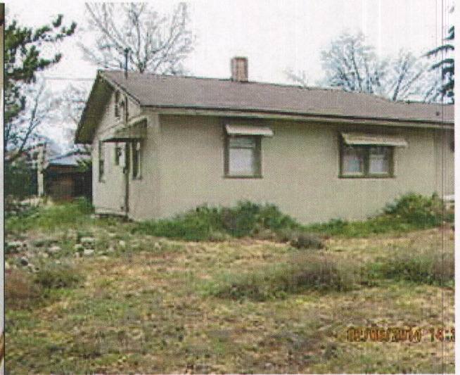
Substandard Structure remains. J. Palmer
