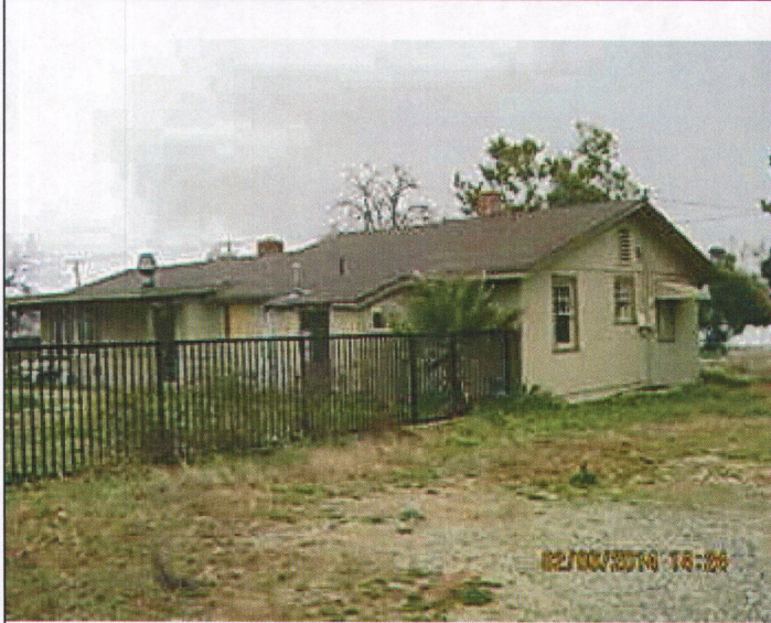
Substandard Structure remains. J. Palmer
