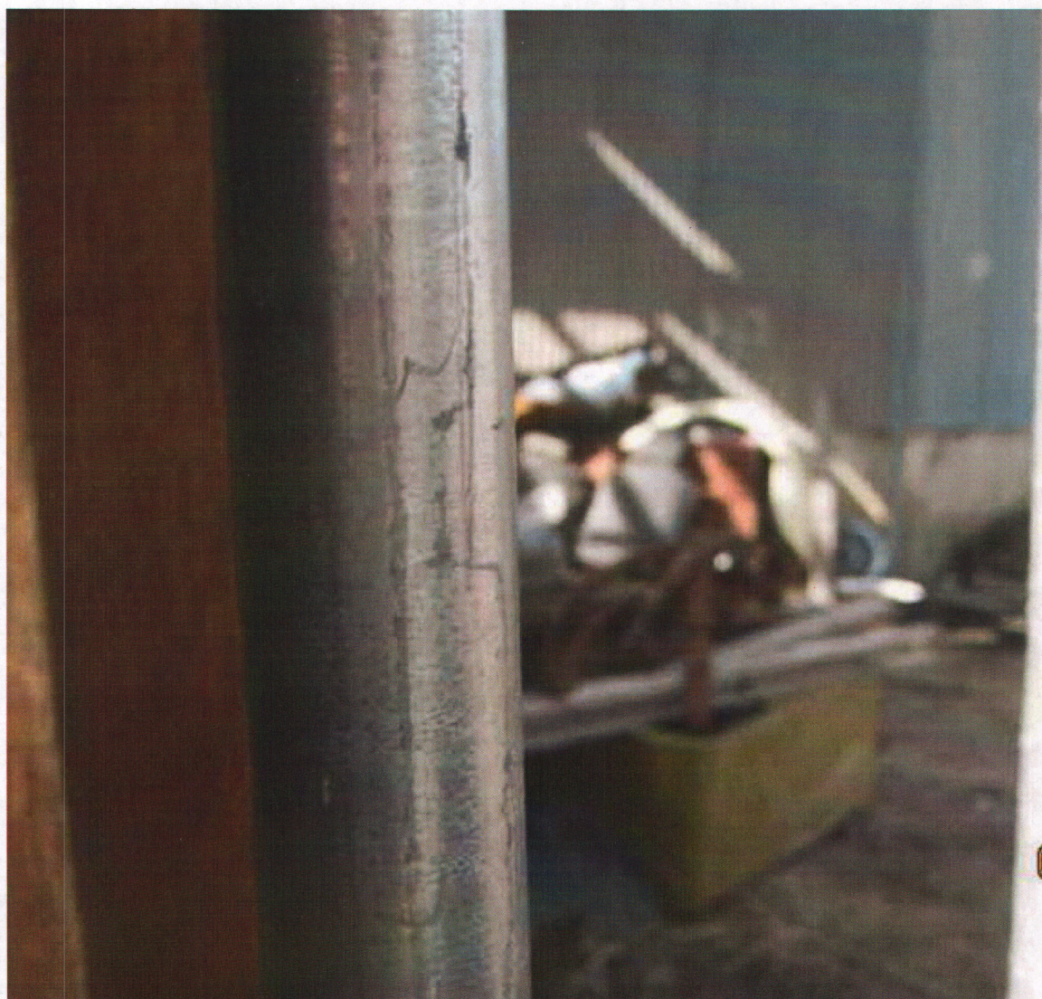
Photo #4 - accumulated rubbish/outdoor storage - 02/04/2014
