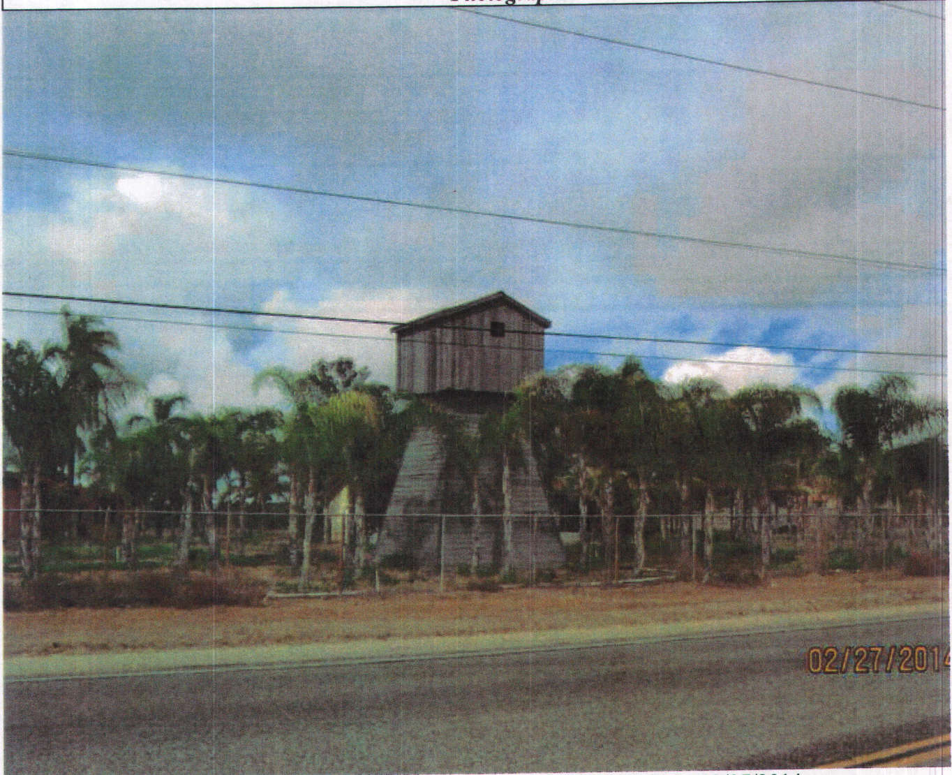
Property remains in violation. Lpadilla 2/27/2014 - 02/27/2014
