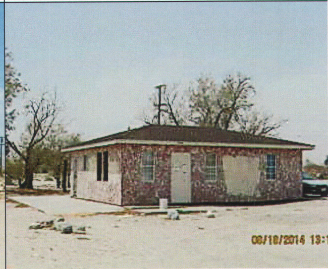
Substandard Structure 8/18/14 J. Cole
