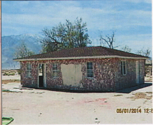
Front of the Structure 5/1/14 J. Cole
