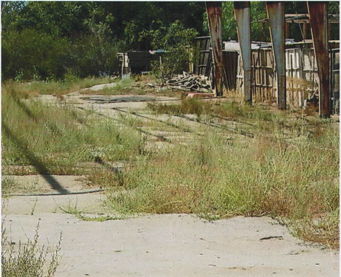
Accumulated rubbish remains-JMorris 8/26/14 - 08/26/2014
