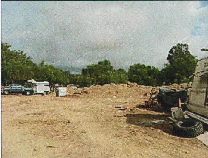
Accumulated Rubbish. Lpadilla 9/26/2013
