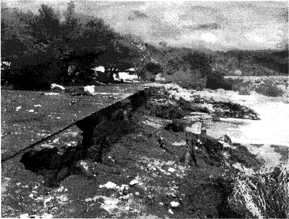
Erosion on banks of the road
