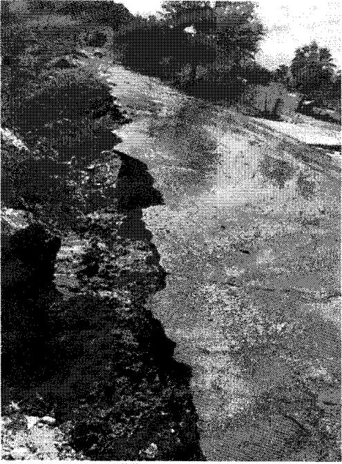
Erosion on banks of the road
