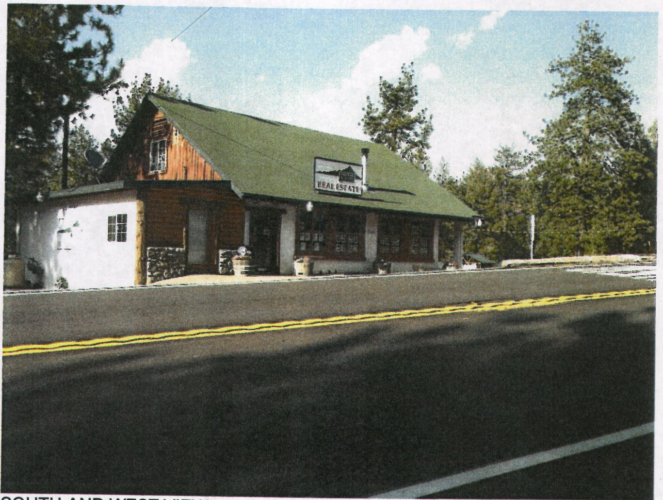
SOUTH AND WEST VIEW
