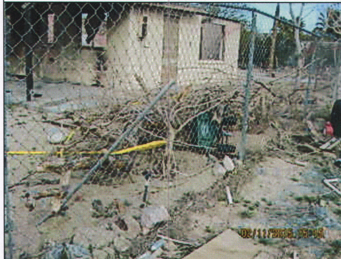
Substandard Structure 2/11/15 J. Cole
