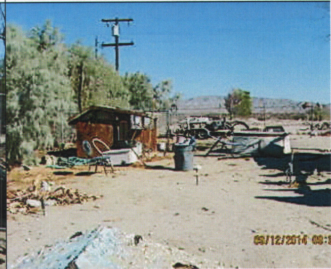
Substandard Structure and Rubbish Remain 9/12/ Cole
