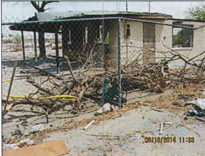
Substandard Structure and Rubbish Remain 8/18/14 J. Cole
