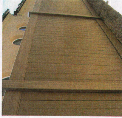
Vinyl Fencing Example
