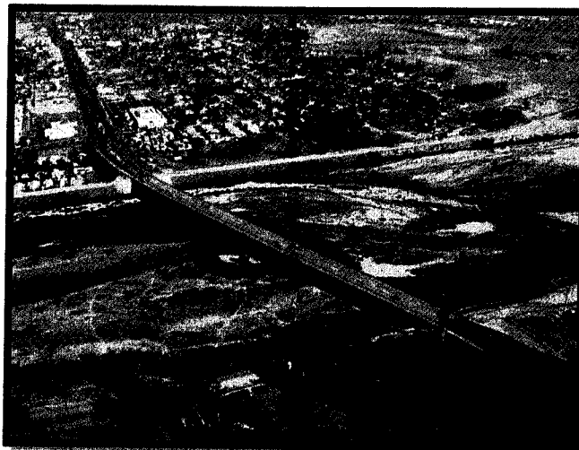
Existing Mission Blvd. Bridge at Santa Ana River (Looking West)
