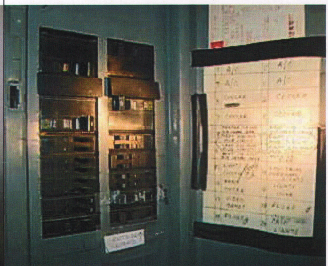
-09/26/14 - Initial Inspection SSST Verified - NC
