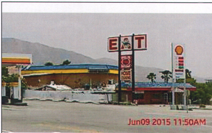
E. Torres; abandoned substandard structure
