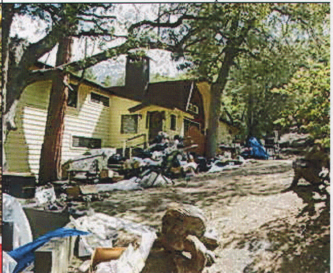
the violation remains with deplorable condition
