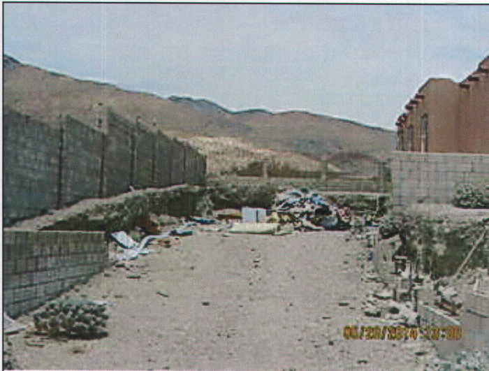
Unpermitted Grading 5/28/14 J. Cole
