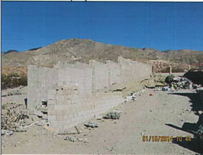
Unpermitted Grading 1/15/14 J. Cole
