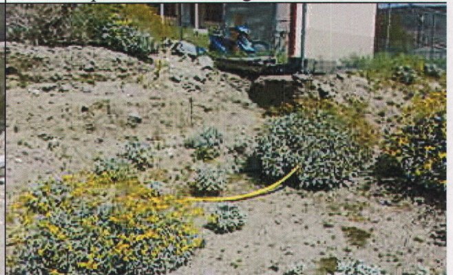
Unpermitted Grading/Cut 3/18/15 J. Cole
