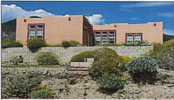
Unpermitted Grading/Cut 3/18/15 J. Cole
