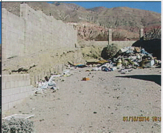
Unpermitted Grading 1/15/14 J. Cole
