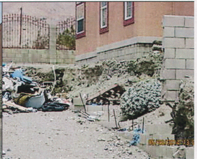
Unpermitted Grading 5/28/14 J. Cole
