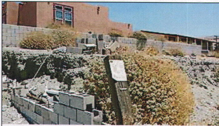
Notice of Violation 7/9/15 J. Cole
