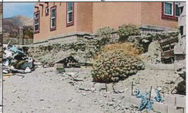
Cut Along the West Side of the Structure 6/29/15 J. Cole
