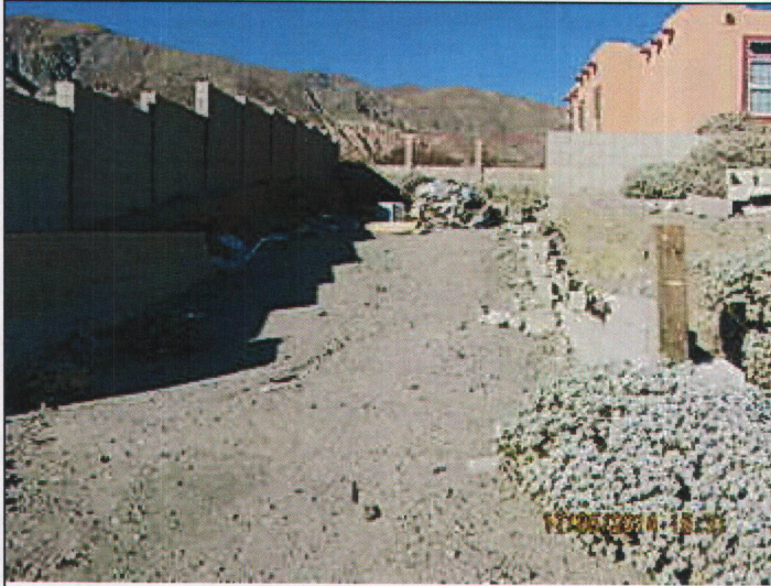
Unpermitted Grading/Cut 11/5/14 J. Cole
