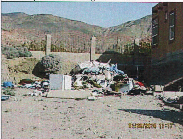
Unpermitted Grading/Cut 1/28/15 J. Cole
