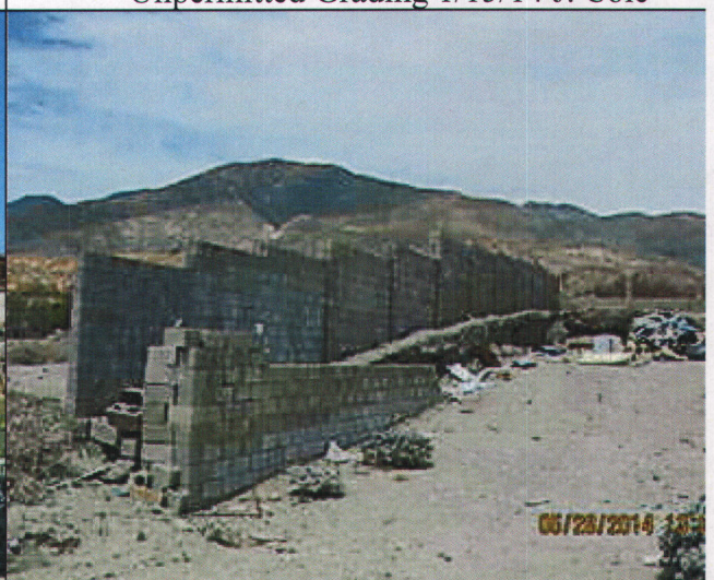
Unpermitted Grading 5/28/14 J. Cole
