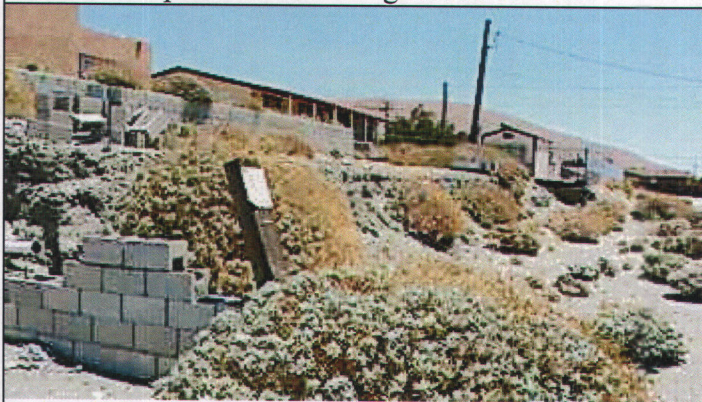
Unpermitted Grading 7/9/15 J. Cole
