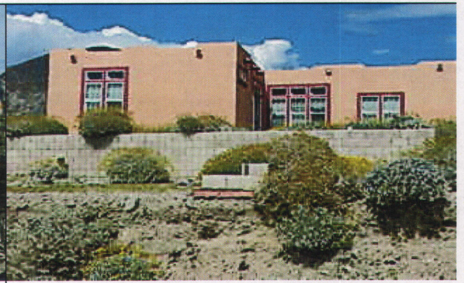
Substandard Structure 3/18/15 J. Cole
