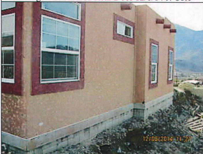
West Side of the Residence 12/8/14 J. Cole
