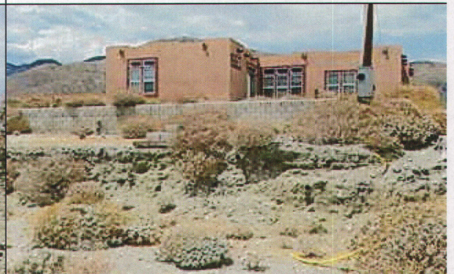
Substandard Structure 6/29/15 J. Cole
