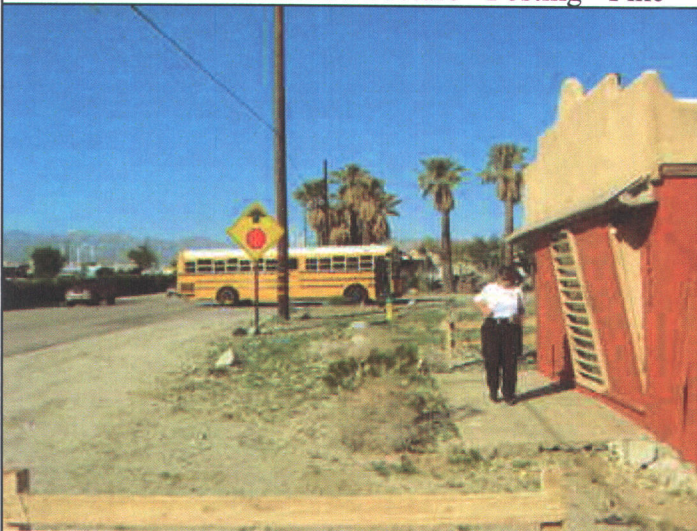
02/05/15 - Substandard Structure - Bus Stop Area - Pike
