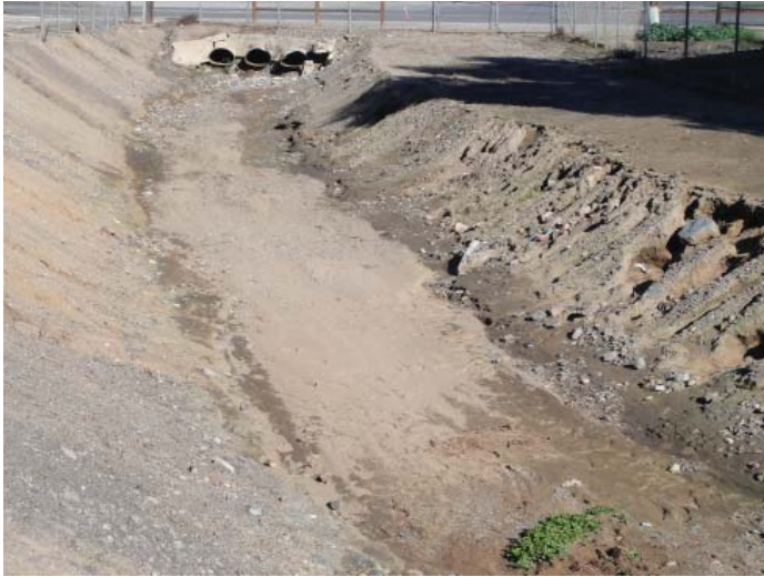
Photograph 5 View east near the Temescal Avenue/ South Norco Channel intersection
