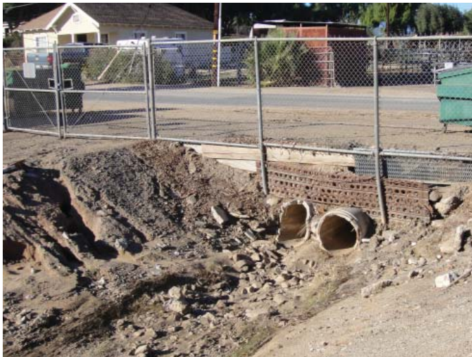
Photograph 3 View north at 3rd Street/South Norco Channel intersection
