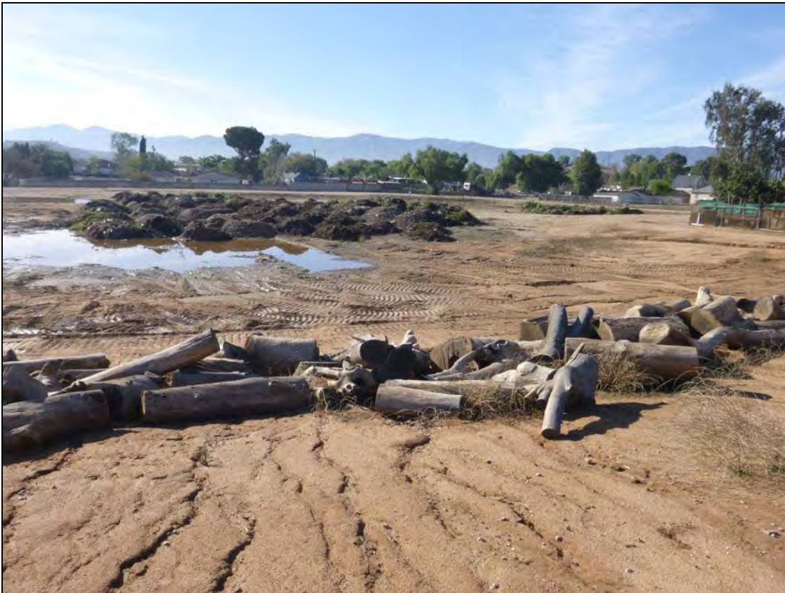
Figure 4-1 View of existing detention basin, facing south.
