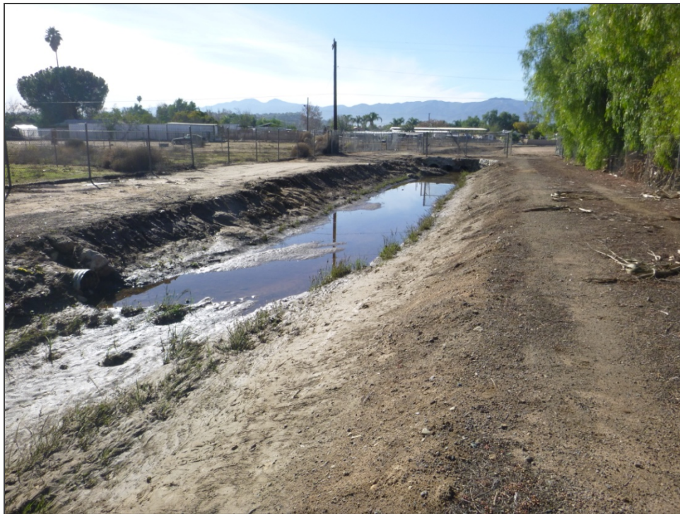
Photo 6-4. Pleistocene age alluvial deposits are completely obscured in the Project area by storm channel construction and grading, vegetation, soil development, recent channel sedimentation, and culvert installation. View to the south.
