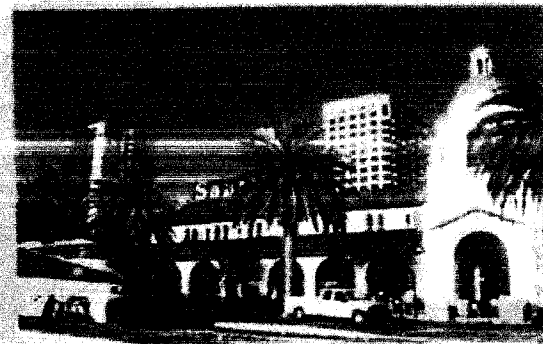
Downtown with Transit Station
