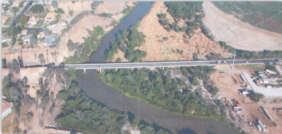
Existing Hamner Avenue Bridge at Santa Ana River (Looking West)
