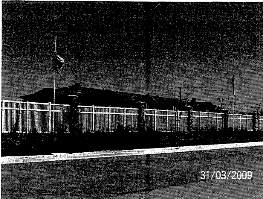
South Side of Property
