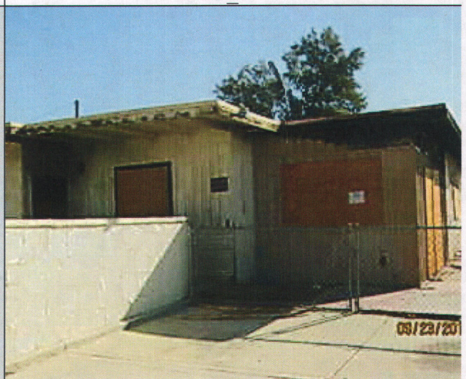
Property remains boarded up and clean. 1 of 2
