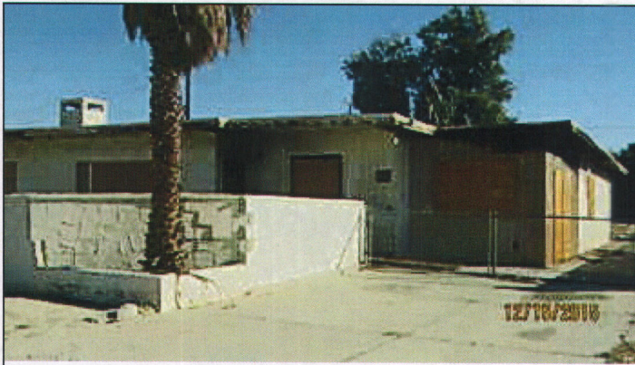
No changes, structure remains boarded up. 1 of 3.
