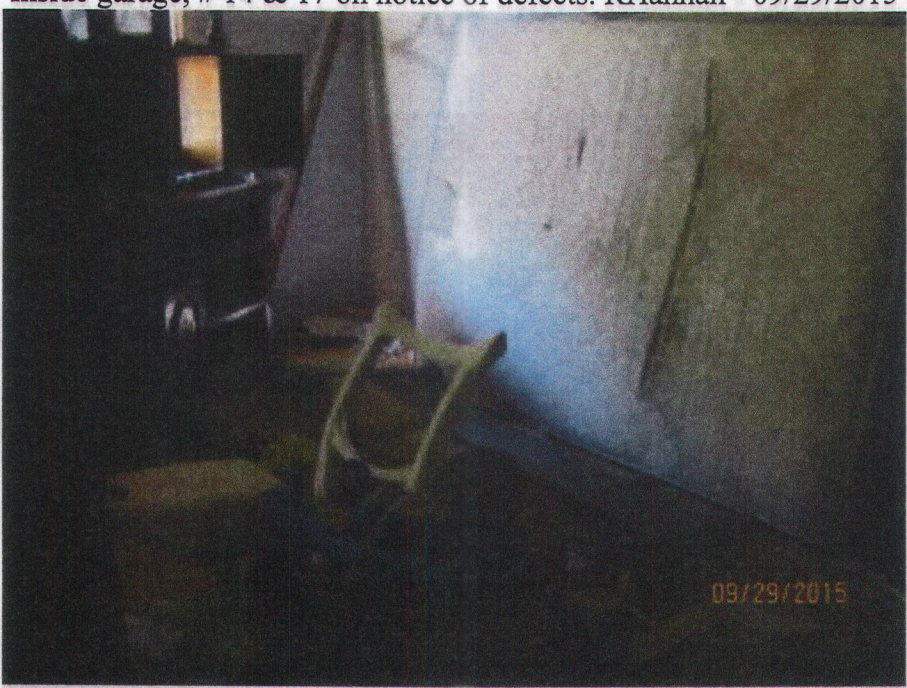
Inside structure. # 14 & 17 on notice of defects. RHannah - 09/29/2015
