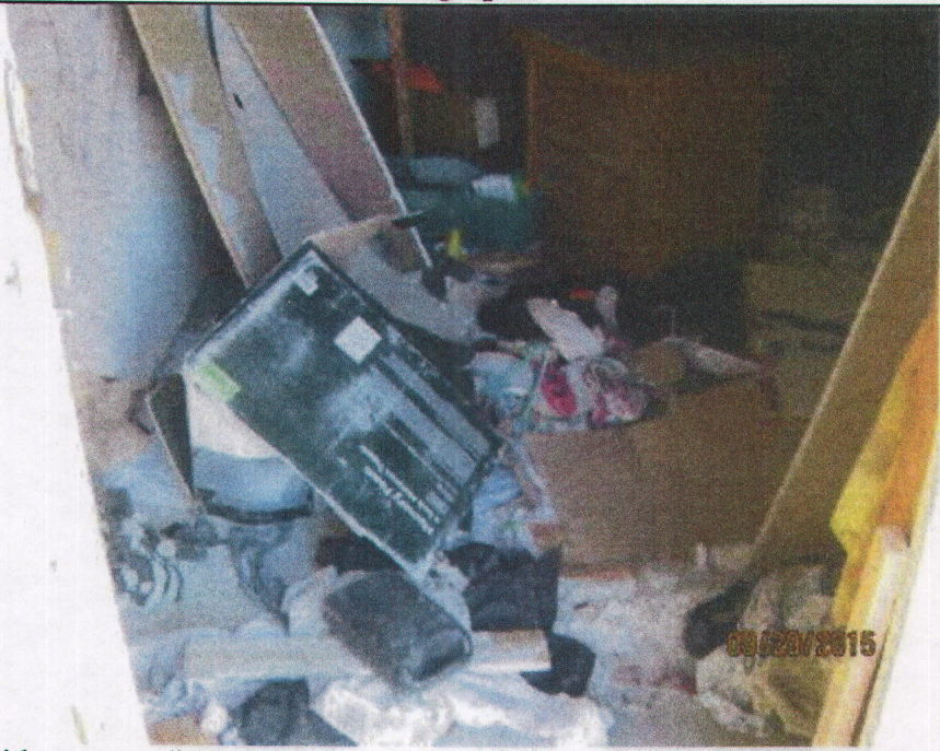
Inside garage, # 14 & 17 on notice of defects. RHannah - 09/29/2015
