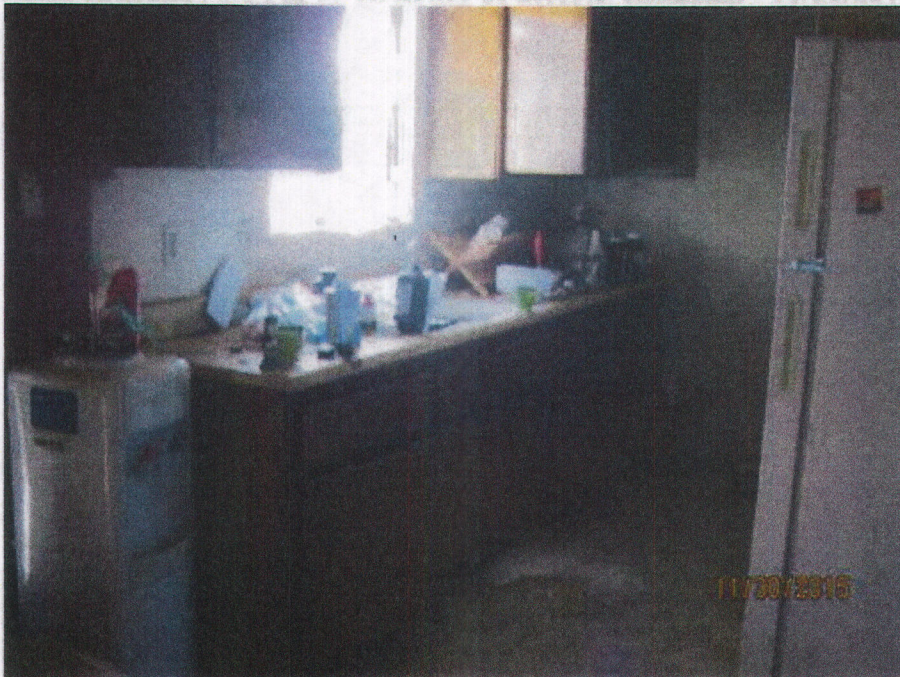
Inside structure'. # 14 & 17 on notice of defects. RHannah - 11/30/2015
