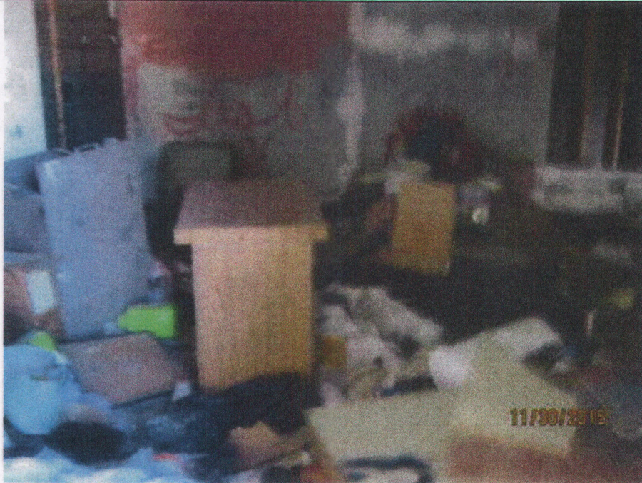
Inside structure'. # 14 & 17 on notice of defects. RHannah - 11/30/2015
