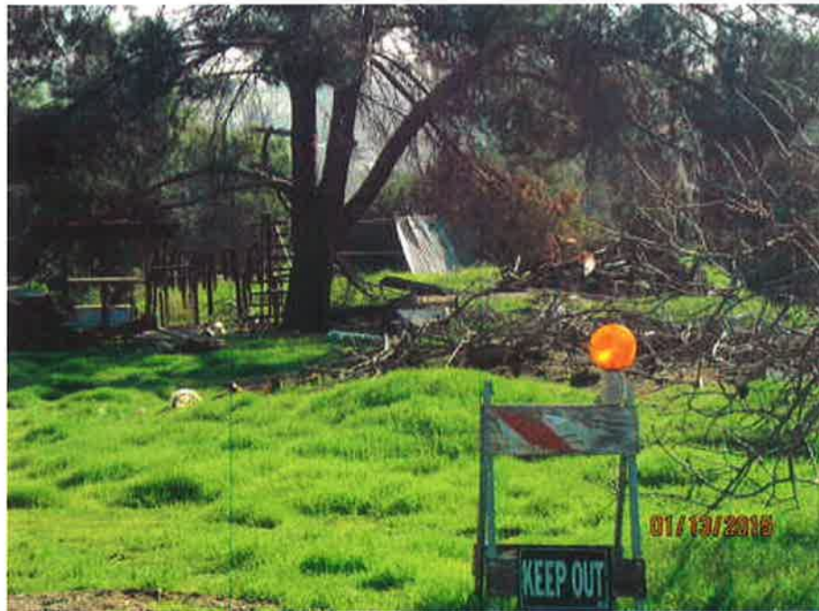
Accumulated Rubbish & Excessive Outside Storage. Lpadilla - 01/13/2015
