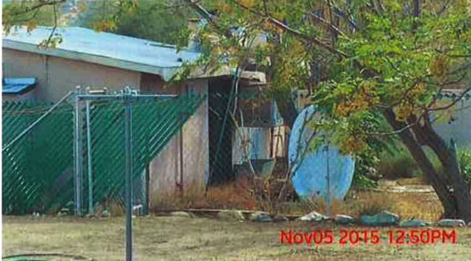
E. Torres; substandard dwelling and AR/EOS in rear yard - 11/05/2015
