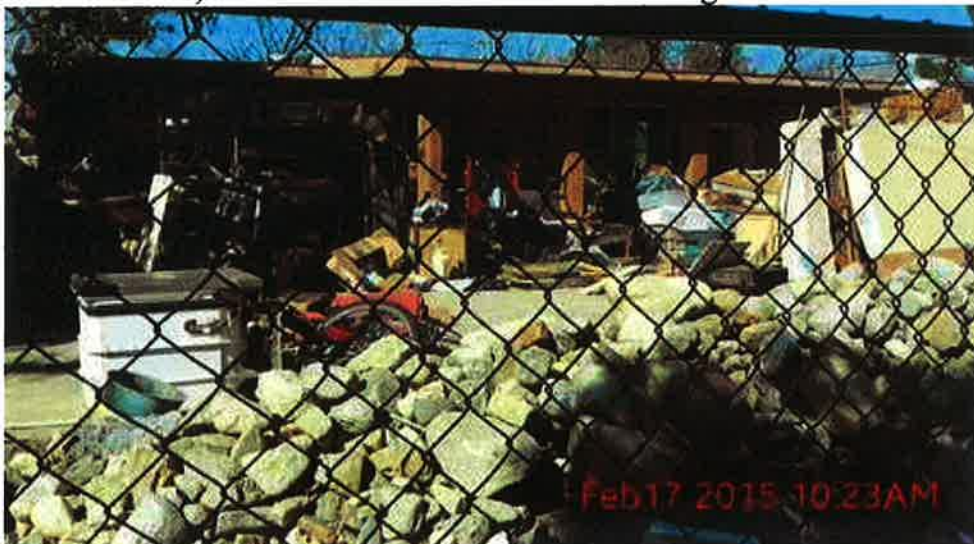
E. Torres; rubbish and excessive outside storage - 02/17/2015
