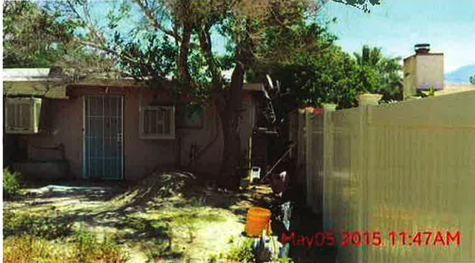
E. Torres; substandard structure #1- defects - 05/05/2015
