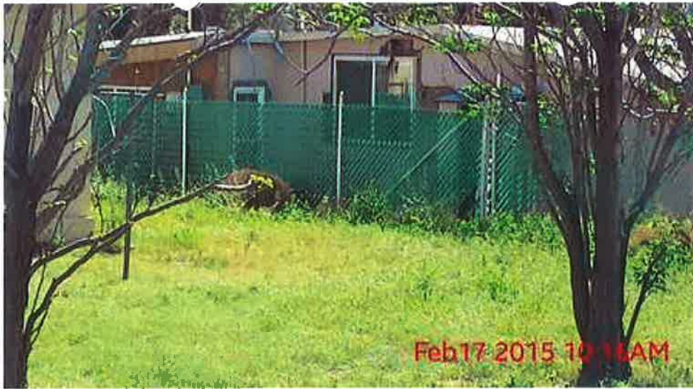
E. Torres; CWP- new electric service panel, windows and door - 02/17/2015
