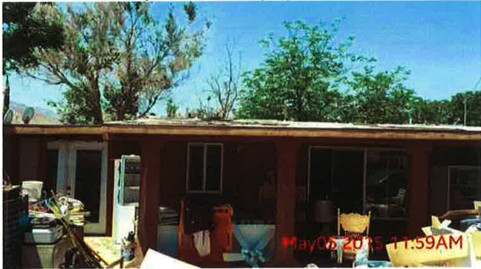
E. Torres; SS1- defects 14, 17, 19 - 05/05/2015
