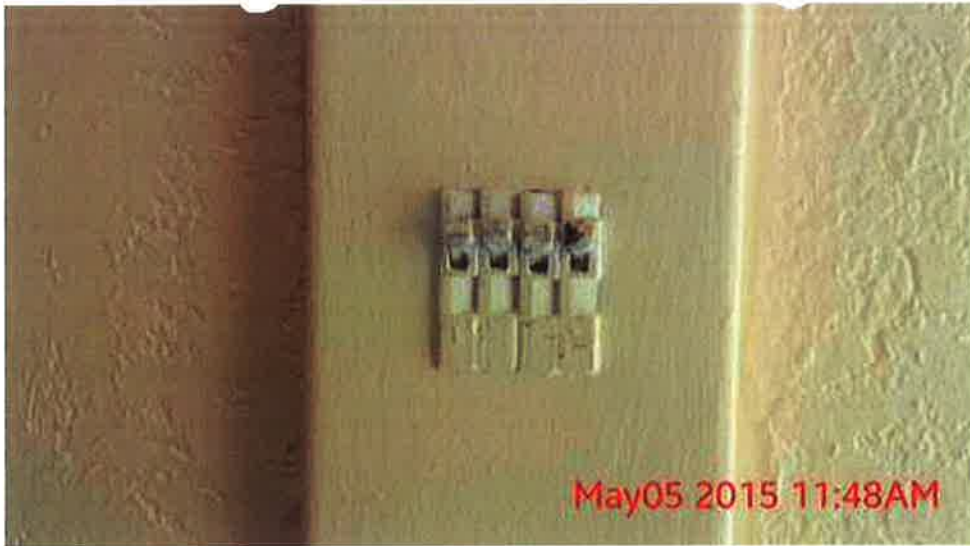
E. Torres; SS2- defects 6, 14, 17, 19 - 05/05/2015
