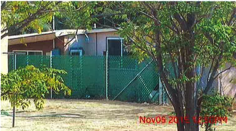
E. Torres; substandard structure- unpermitted electric service panel replacement - 11/05/2015
