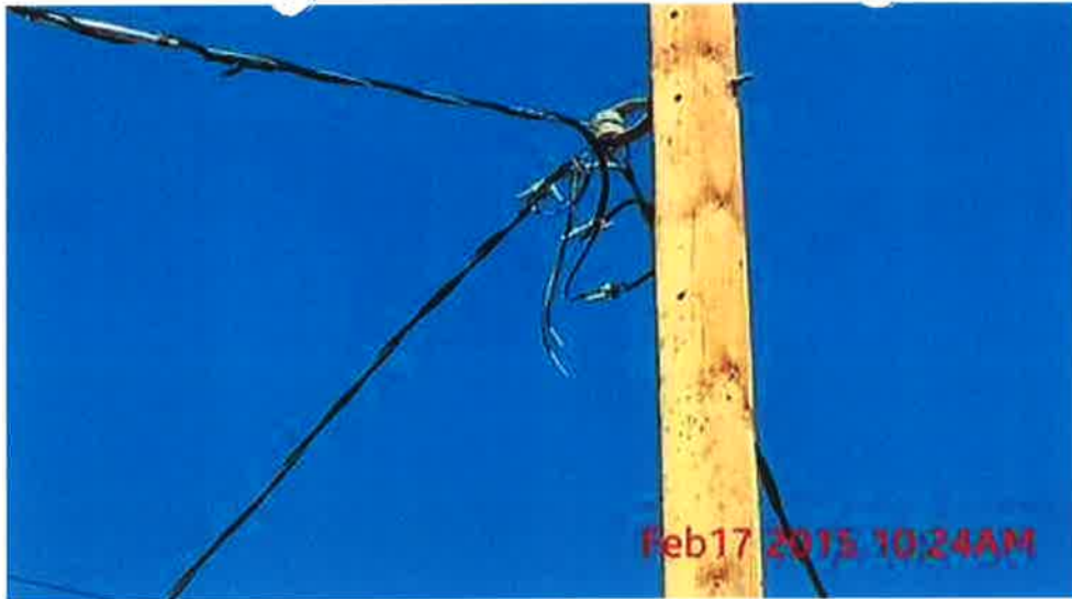
E. Torres; power to property pulled by Edison - 02/17/2015
