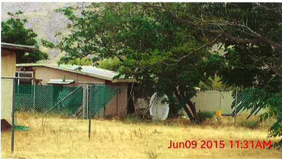
E. Torres; view from road- rear yard - 06/09/2015
