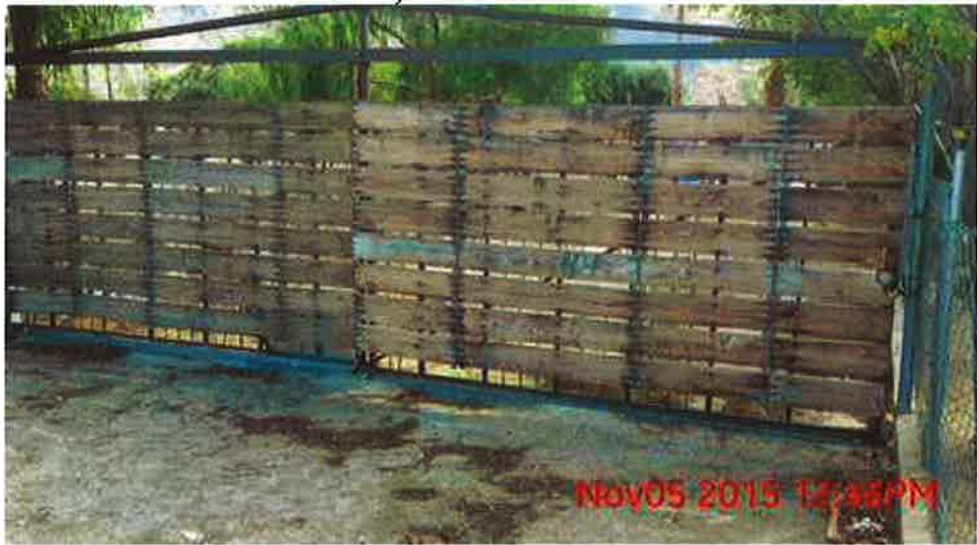
E. Torres; front gate repaired - 11/05/2015
