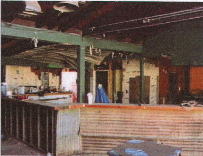
110215 TM stripped interior
