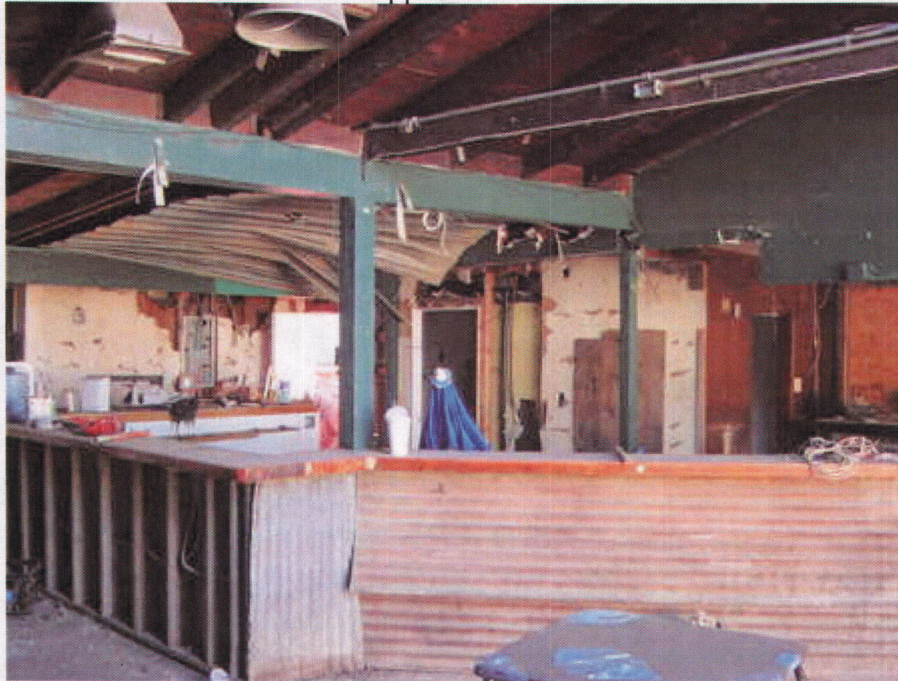
110215 TM stripped interior - 11/03/2015
