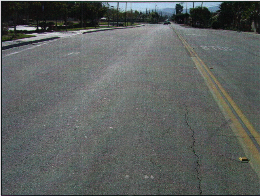
Figure 11C. PCI=78 (Good Condition)
