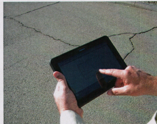
Figure 15. Tablet device use in road inspection.
