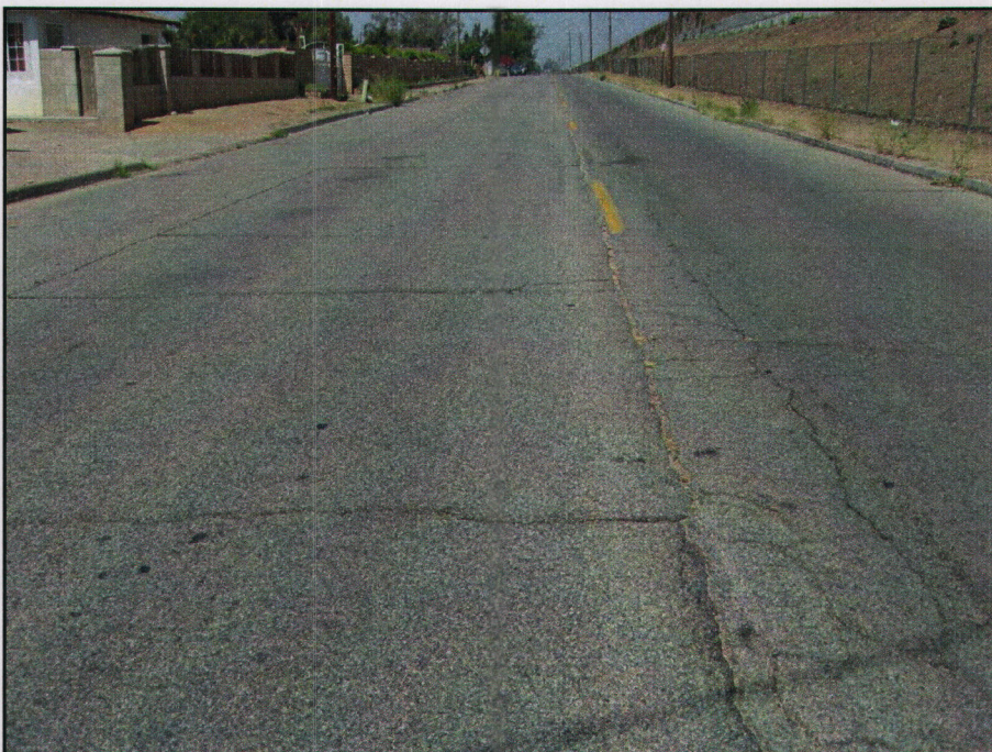
Figure 11D. PCI=56 (At Risk Condition)
