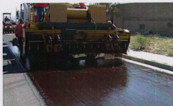
Figure 19. Spreading of chip over emulsion.
