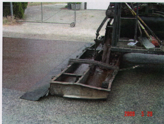
Figure 20. Spreading of slurry.
