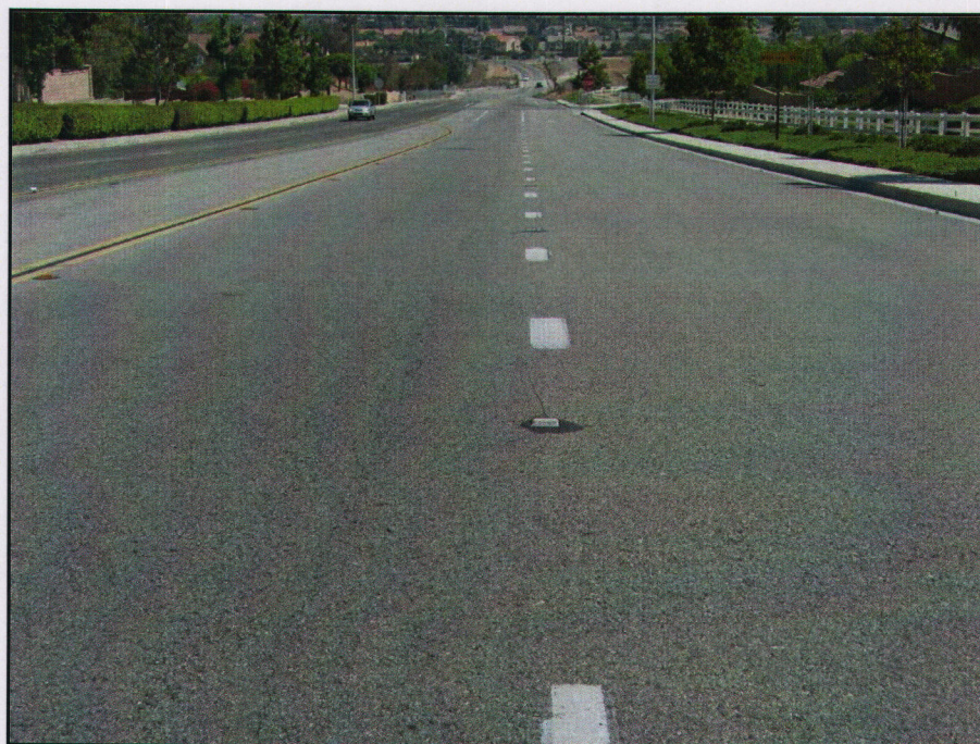
Figure 11B. PCI=85 (Very Good Condition)
