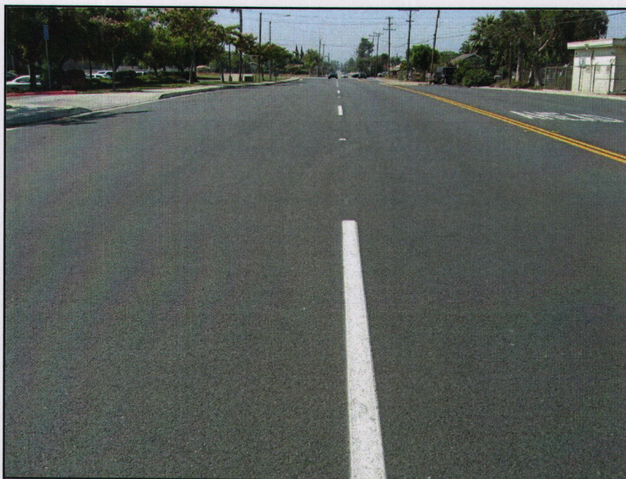
Figure 11A. PCI=98 (Excellent Condition)
