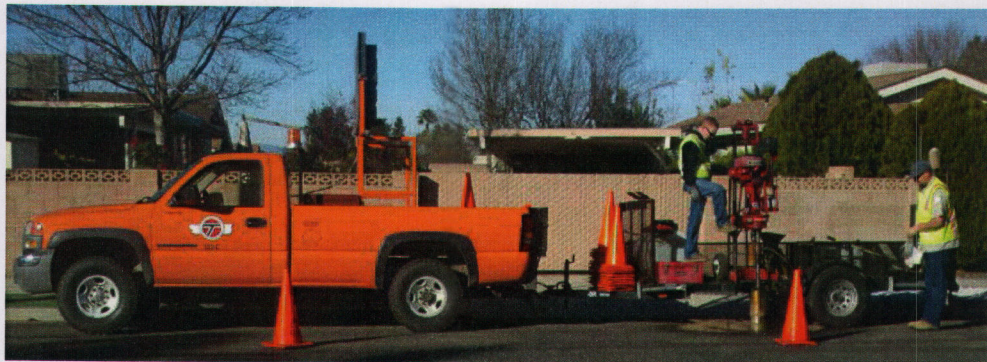
Figure 17. County's Coring Rig
