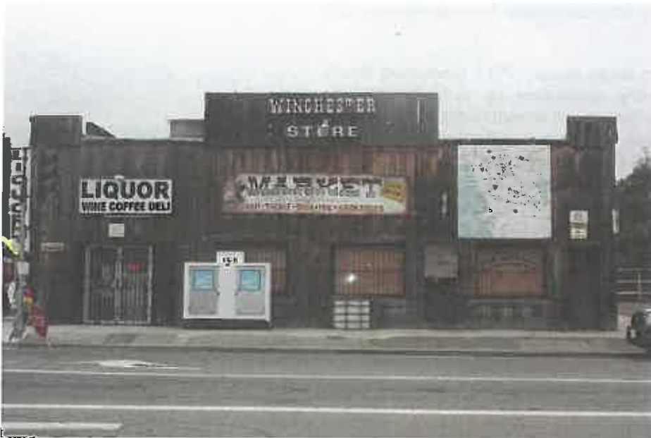
Existing Commercial Building
