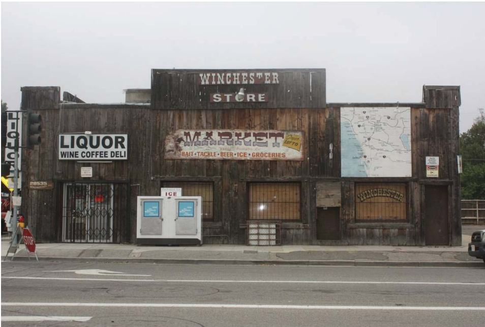
Existing Commercial Building
