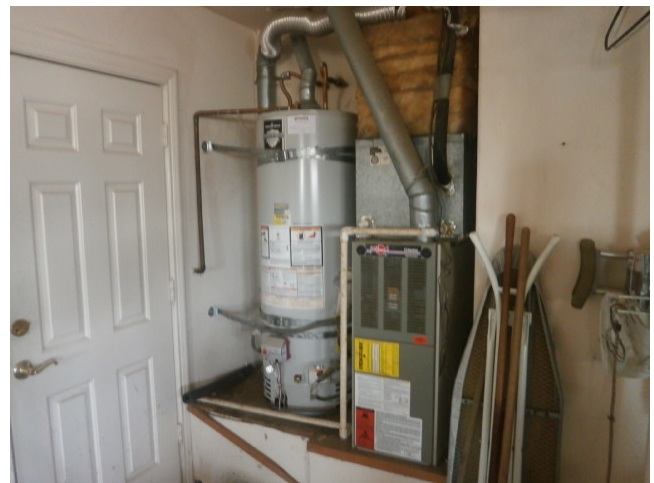
Water heater and furnace
