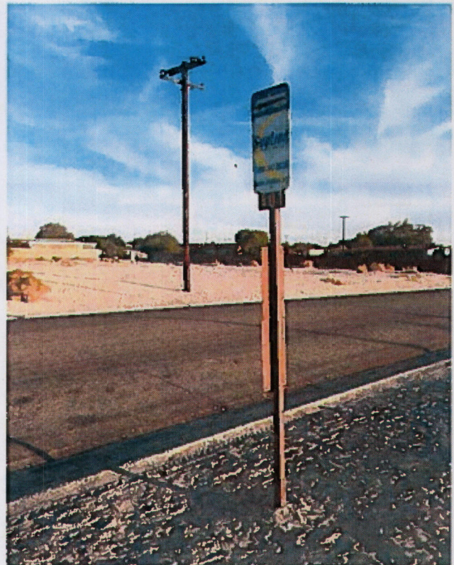
North Shore — Miramar Drive: Sunbus stop with no shade structure or bench.
