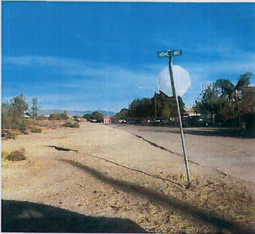
Mecca — Corner of 5 th Street and Home Avenue: No sidewalks or safe and clean path for pedestrians.
