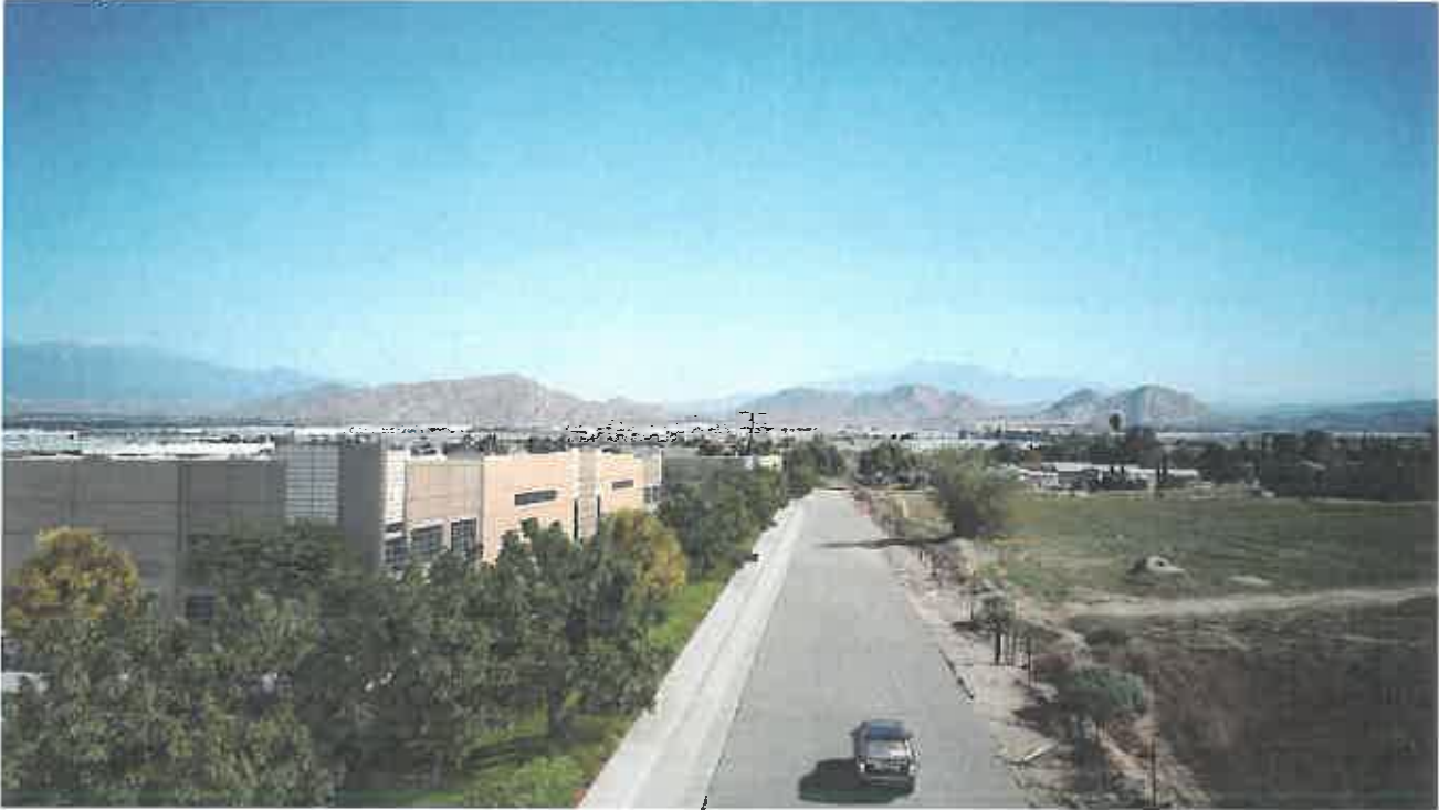
Building E Southern Boundary Viewed from the West
