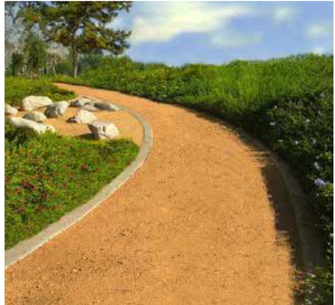
example of a stabilized DG trail
