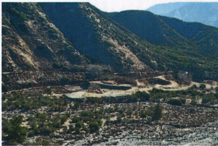
Surface water diversion spreading basins along the San Gorgonio River located within Banning Canyon
