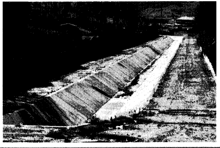
Local flood control channel
