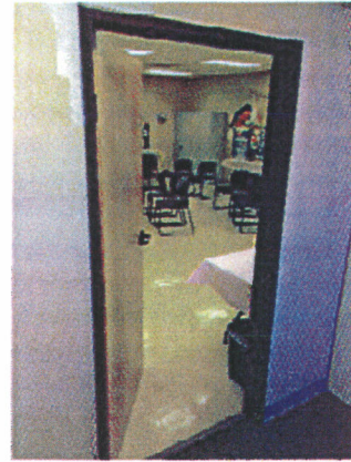
Secondary Classroom 1 entrance door
