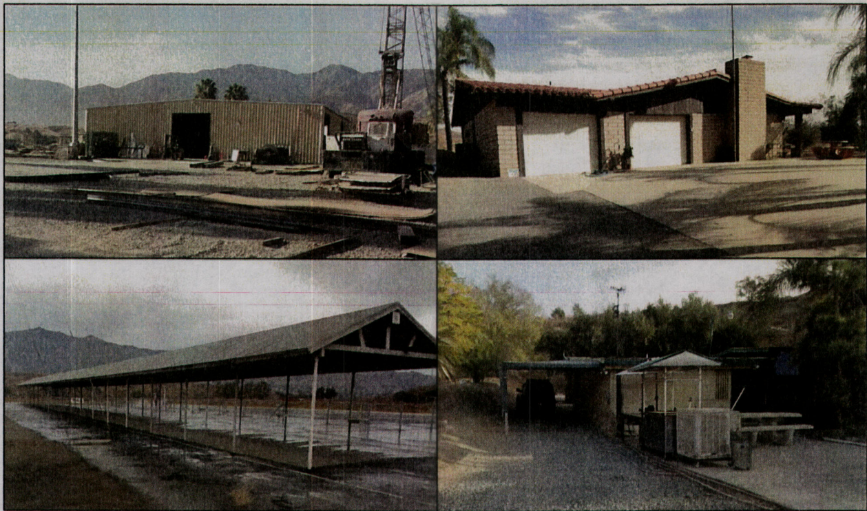
Figure 7. Representative buildings in the project area. Clockwise from top left : storage building; caretaker's residence; office/employee lounge; shade structure at the model airplane field. (Photographs taken on November 17 and 20, 2017)
