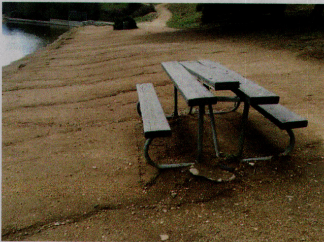
A picnic table in need of repair.
