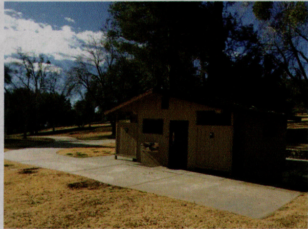
A restroom in good condition.
