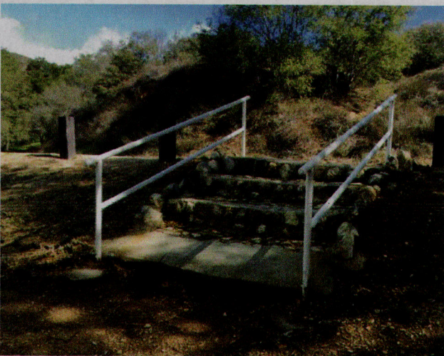
The base of the landing requires fill soil.
