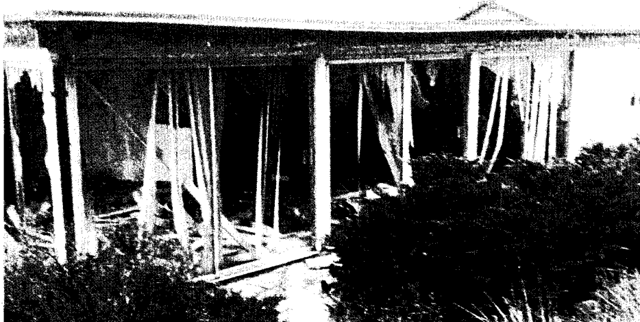
Condition of Ranch house February 2018.
