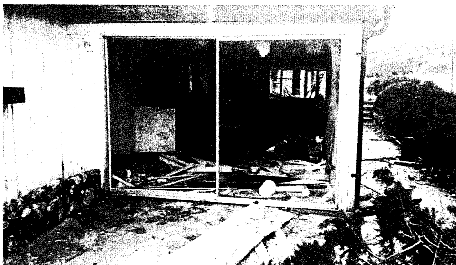
Condition of Ranch house February 2018.
