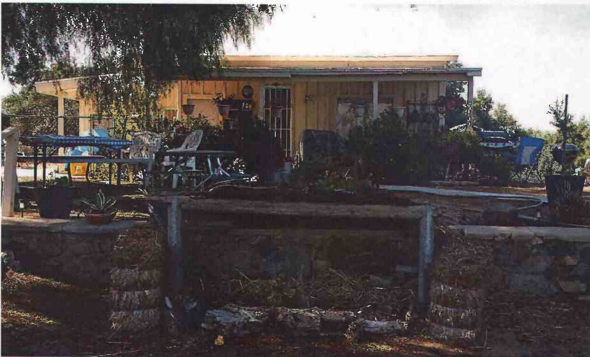
Photo # 26 Front of residence.
