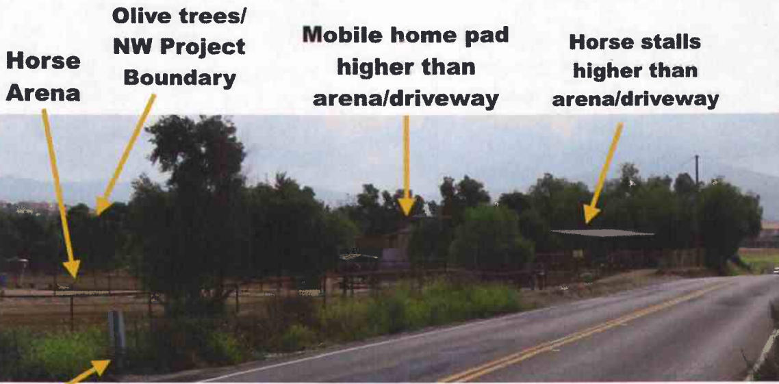
Reflector marking Culvert that directs storm water from S of Los Alamos Road to the N, towards NW boundary of Project
