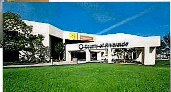
Rustin Conference Center – Riverside, CA
