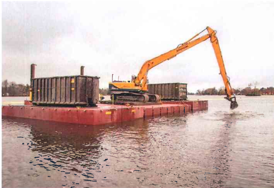
Figure 5 Typical Barge Mounted Excavator w/ Bucket
