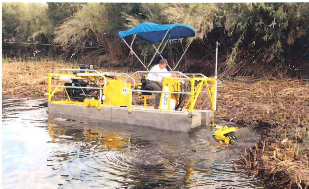
Figure 3 Typical Hydraulic Dredging Barge 2
