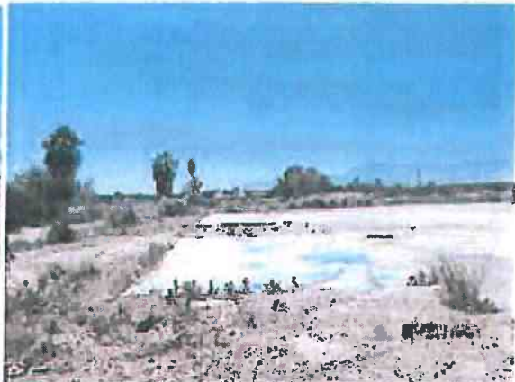
Photo #2 - Looking south from NE corner
