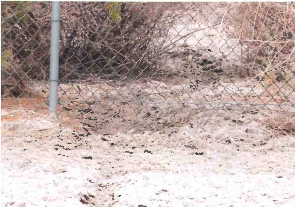
Photo 9: Evidence of burrowing beneath the perimeter fence by coyotes and dogs. The burrows and holes provide access to the AOA.
