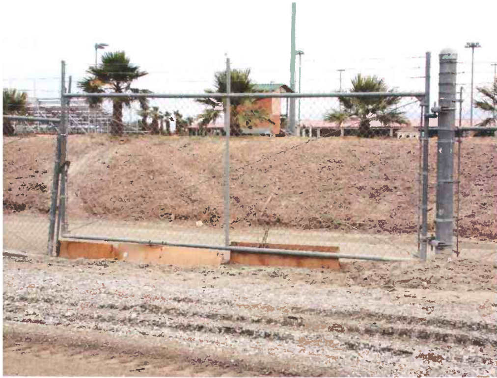
Photo 10: Some gaps beneath the perimeter fence gates have been addressed, but these temporary repairs are not successful at excluding coyotes and dogs.
