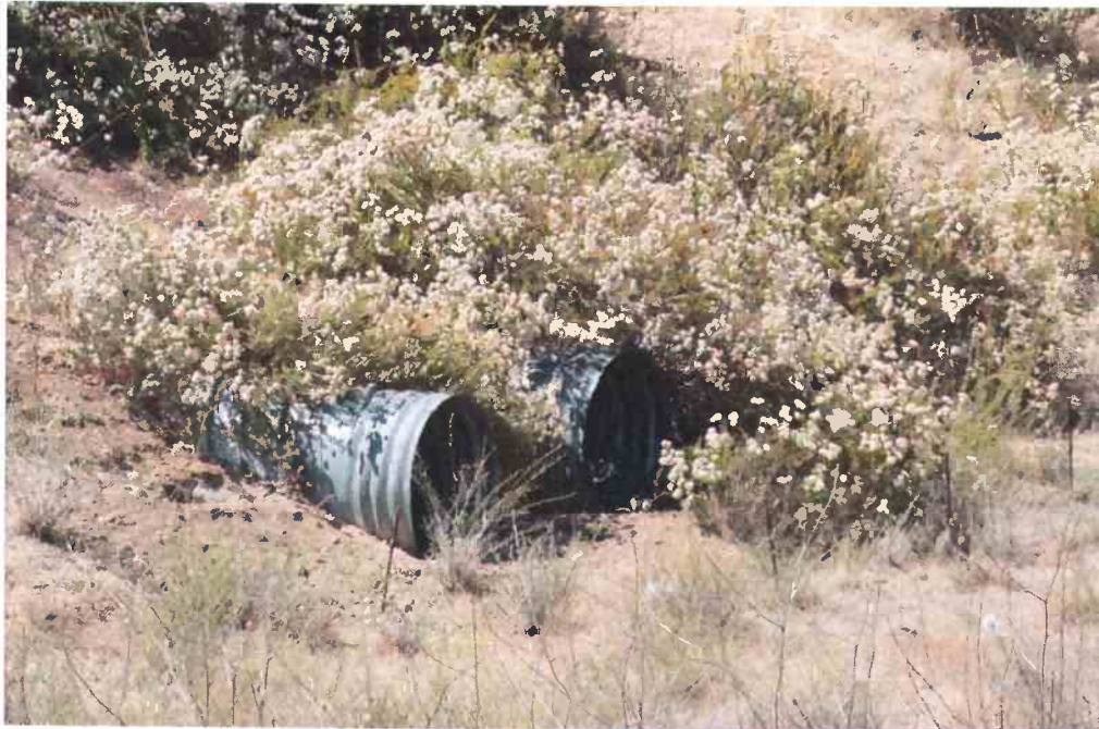
Photo 6: Culverts with open ends allow coyotes and other mammals to enter the AOA.
