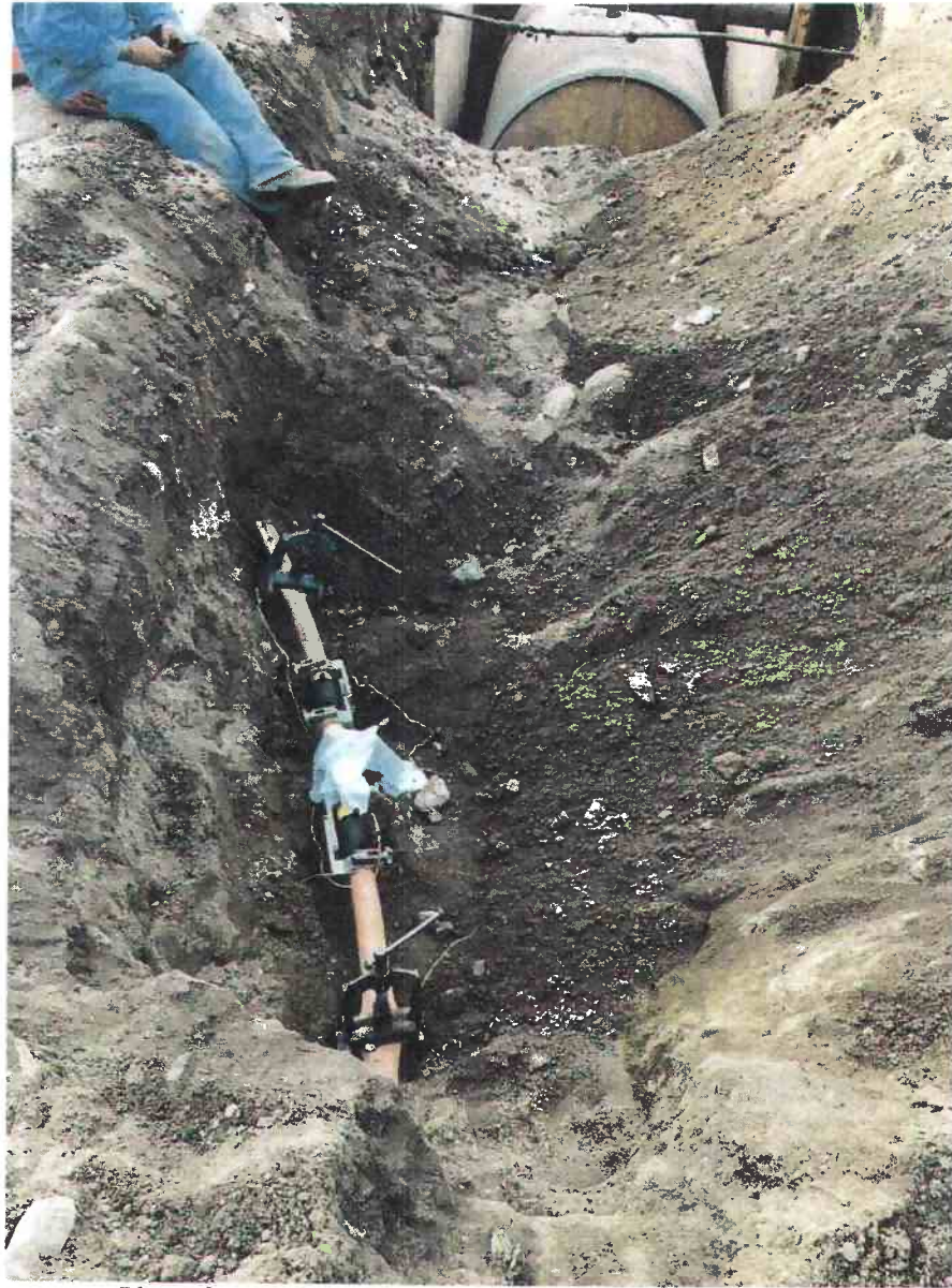
Photo 2 - Gas Line Repaired in Storm Drain Alignment
