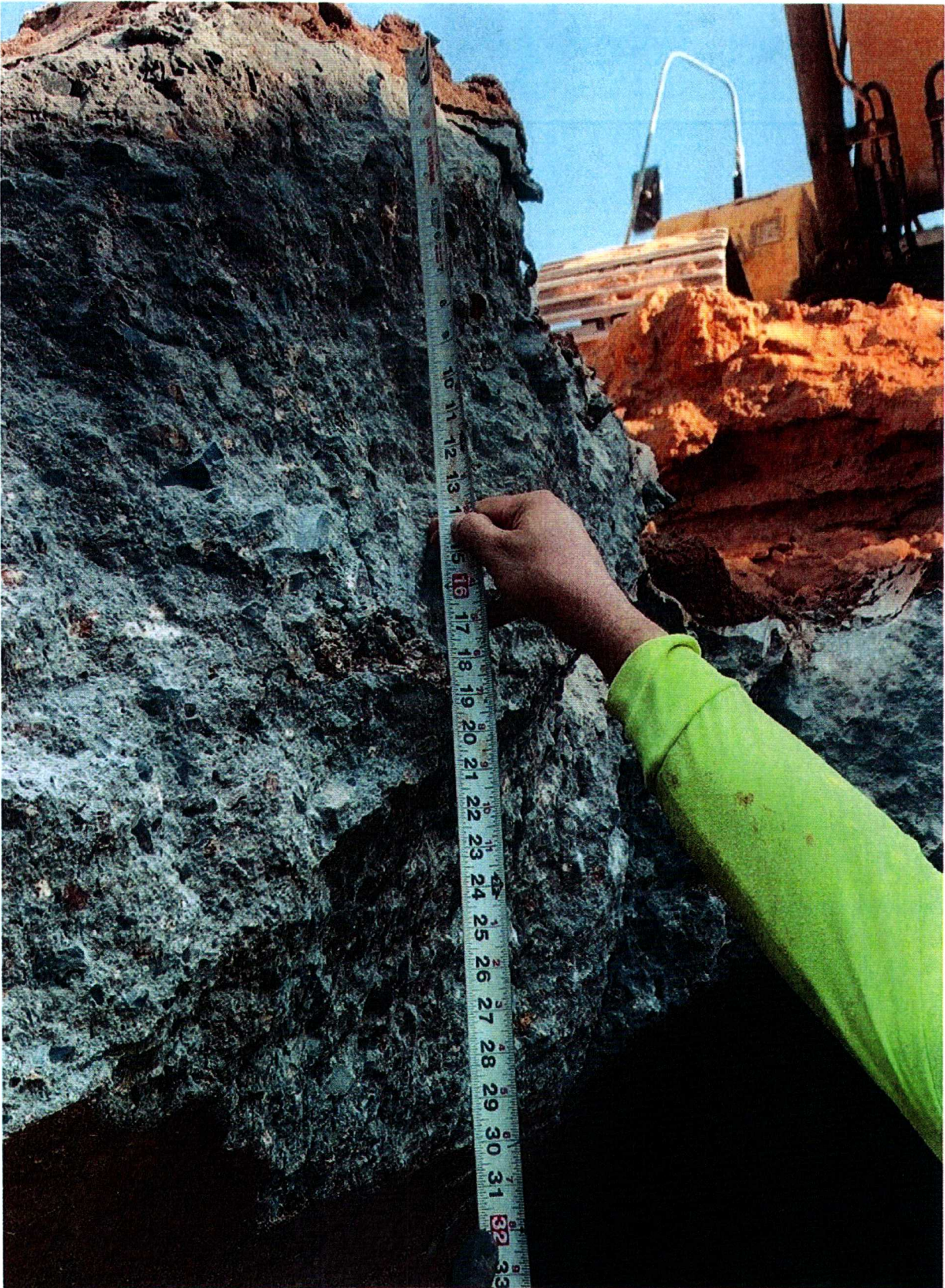
Photo 2 - Existing CIPP measurement
