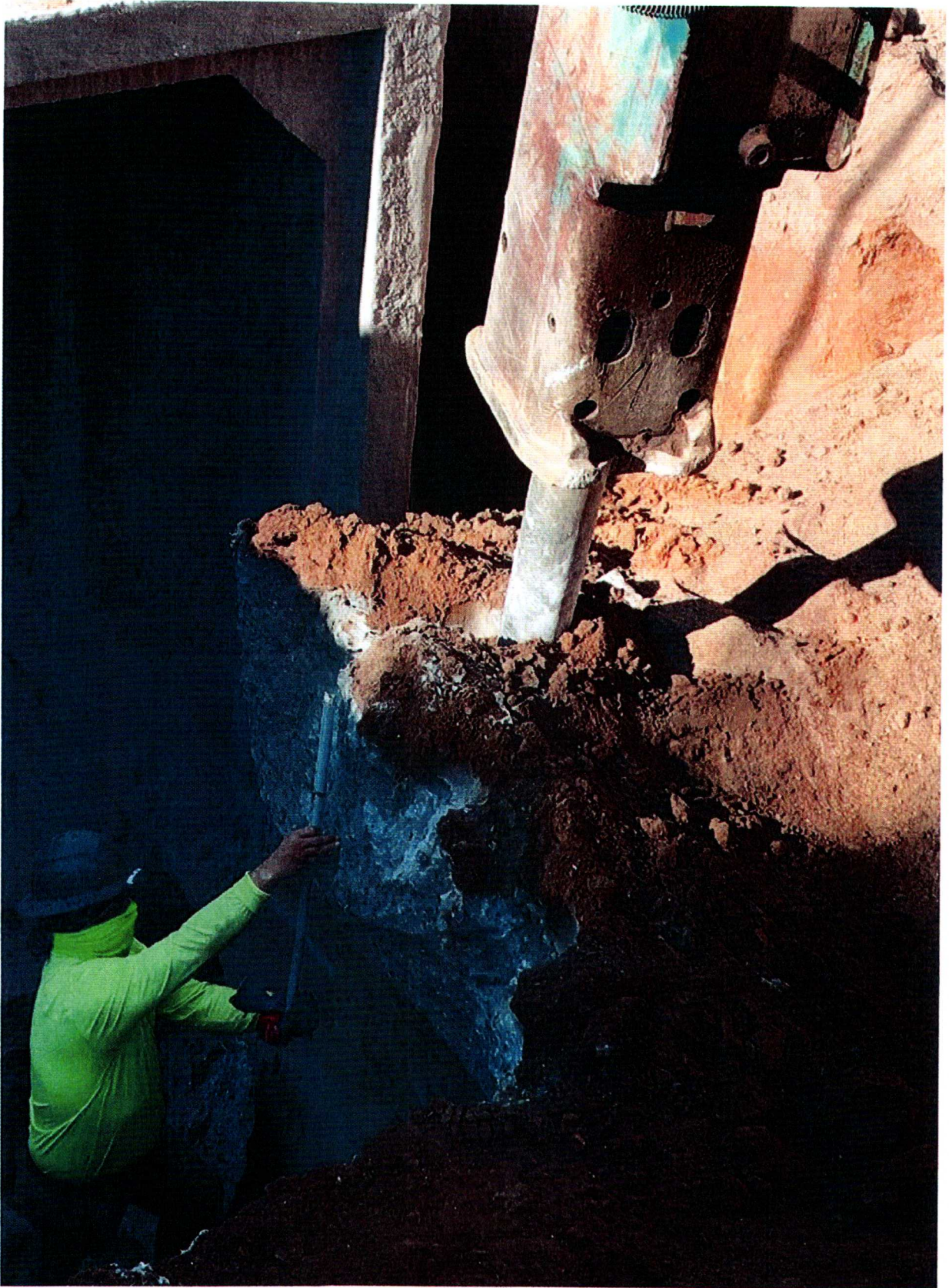
Photo 1 - Construction worker measuring existing CIPP and 10,000 LB breaker
